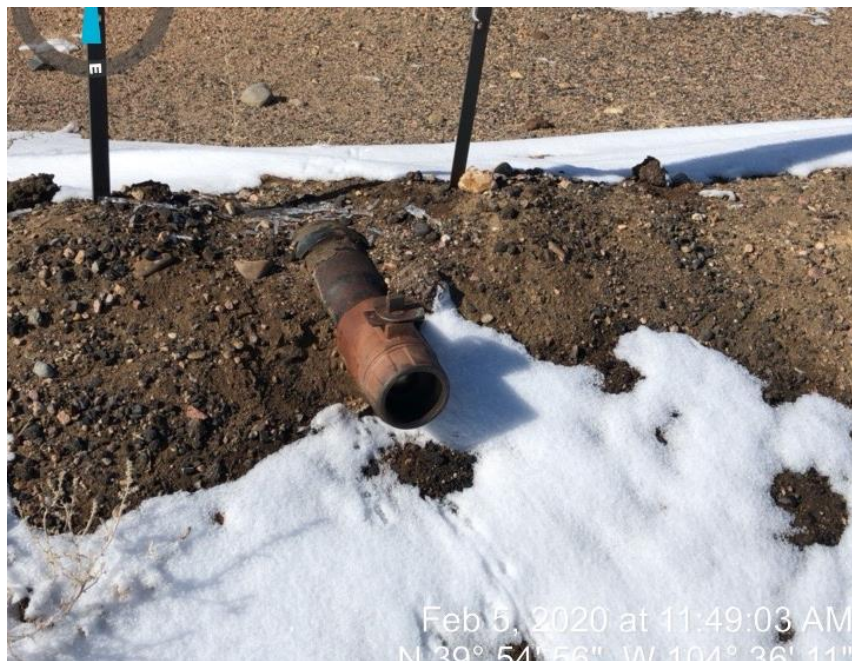
Photo #7 load off line with no bull plug
