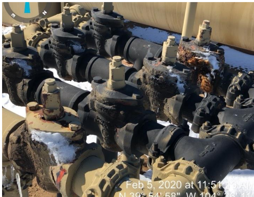
Photo #9 leaking valves
