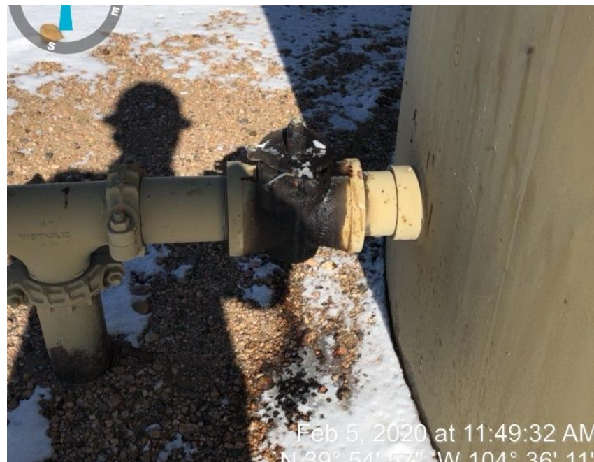
Photo #8 leaking valve and stained soil
