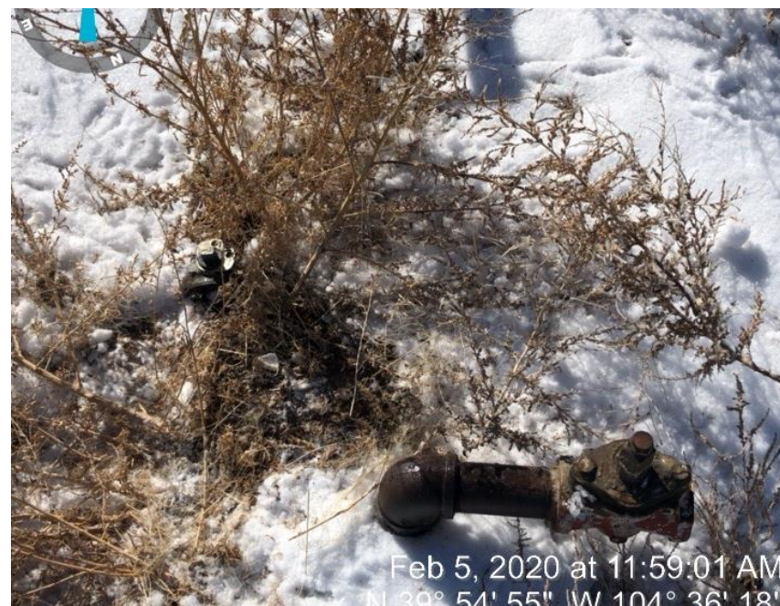
Photo #12 unmarked risers by pumpjack
