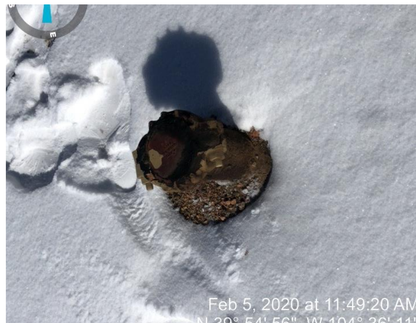
Photo #6 unmarked riser south of crude tank
