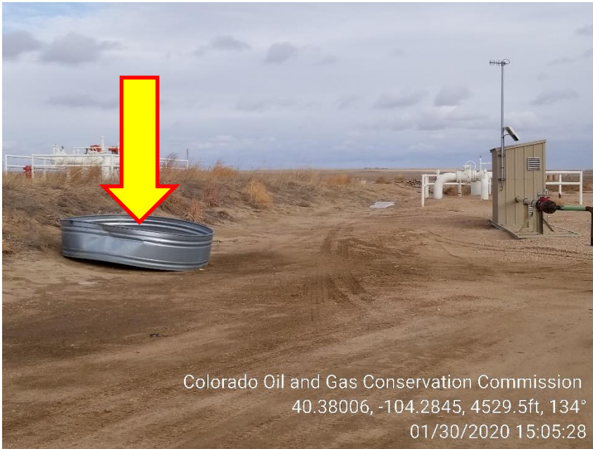
Photo 3 – Unused Secondary Containment
