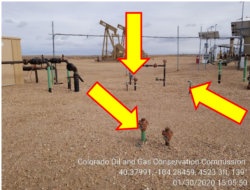
Photo 1 – Unmarked Riser North of Heater Treaters
