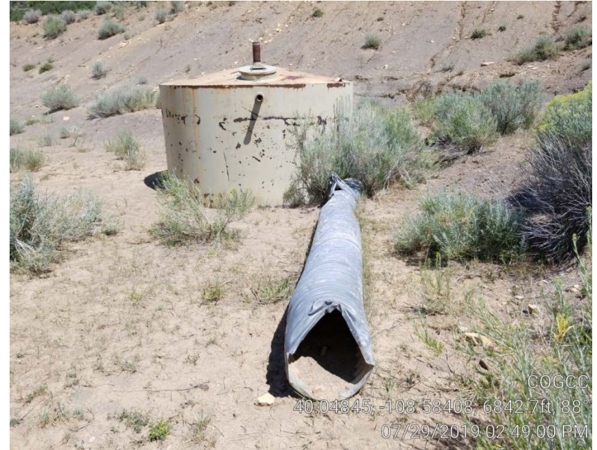
Photo 15. Damaged culver on 7-29-2019.
