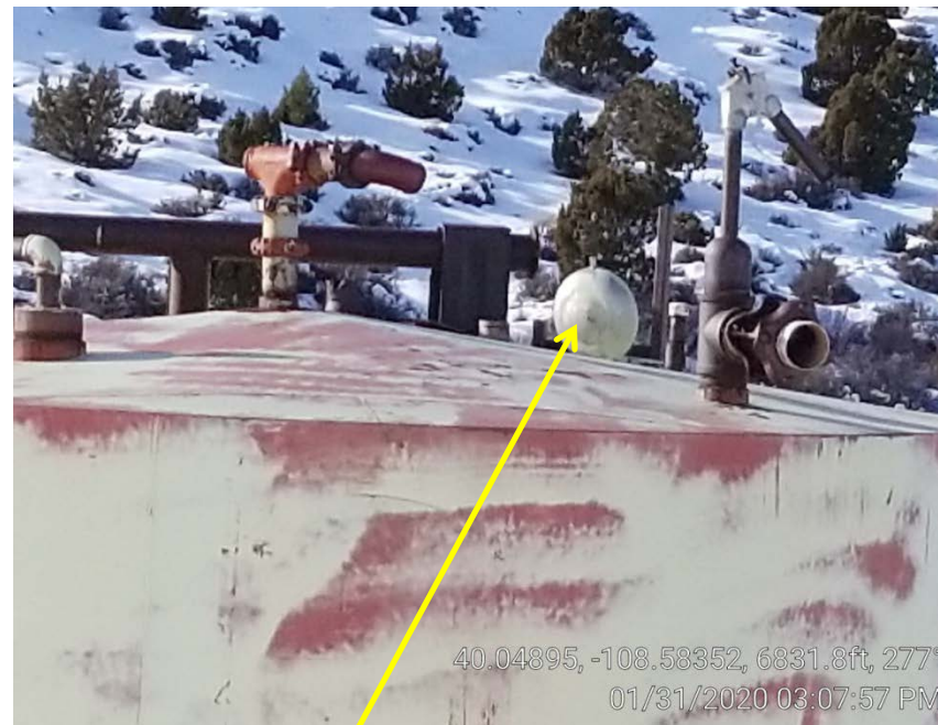
Photo 19. Open tank hatch on portable tank.
