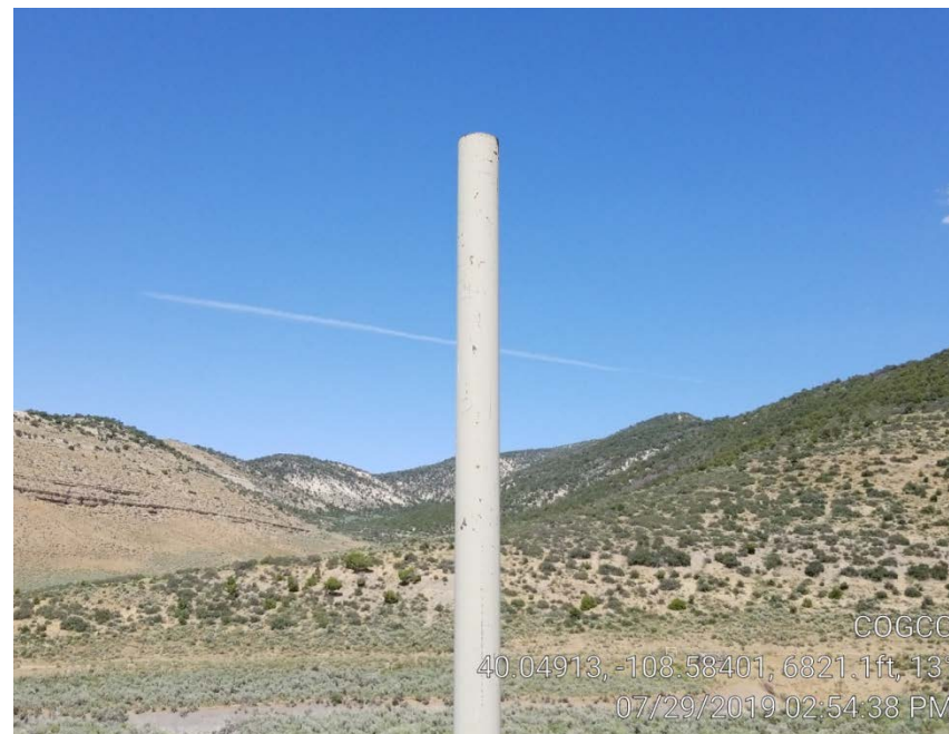
Photo 9. No apparent bird screen on tank vent on 7-29-2019.
