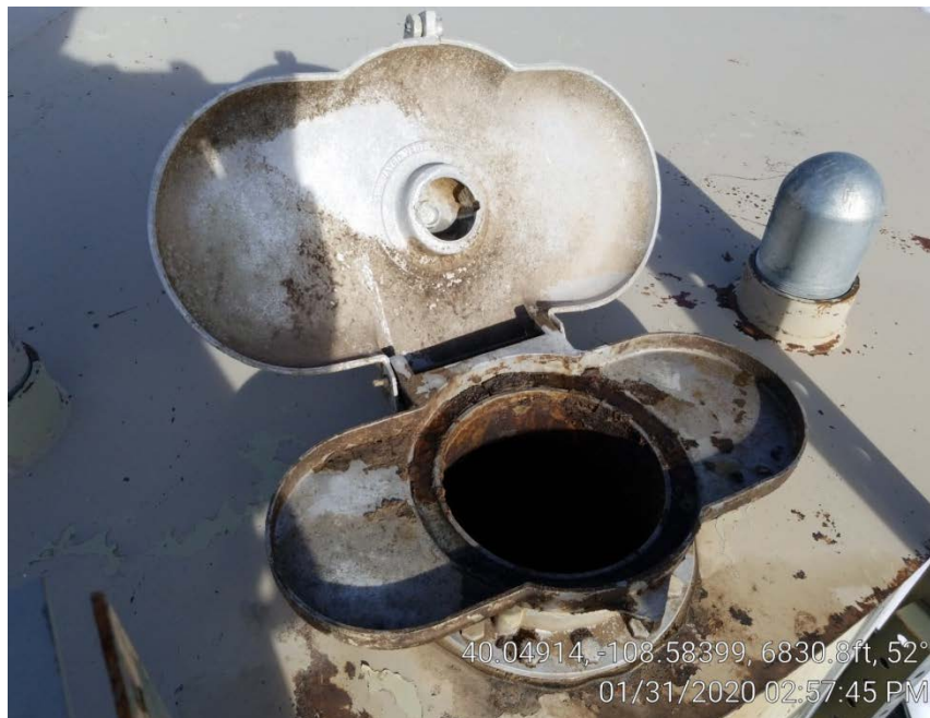
Photo 18. Open tank hatch on permanent tank.
