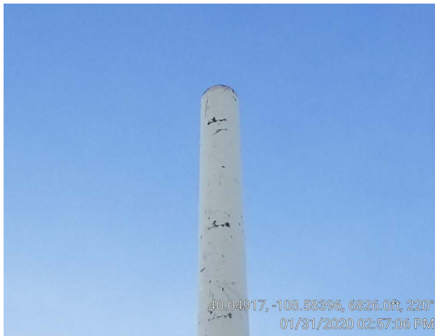
Photo 8. No apparent bird screen on tank vent on 1-31-2020.
