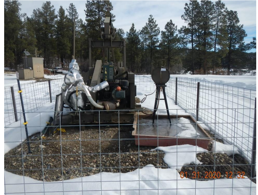
Secondary containment for lube oil container is almost full of ice.
