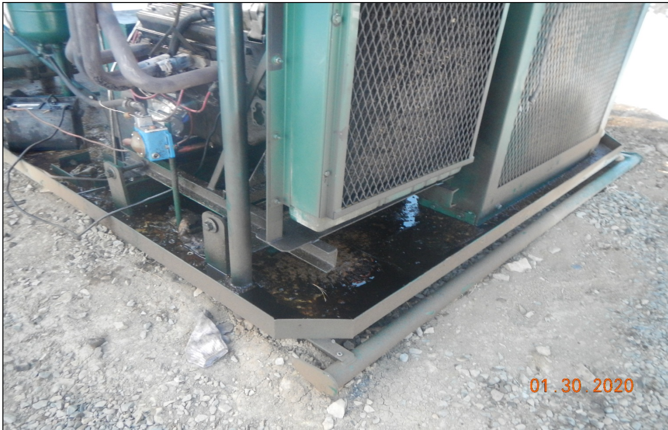
Photo 4. There is oily waste at the engine skid at the separator.
