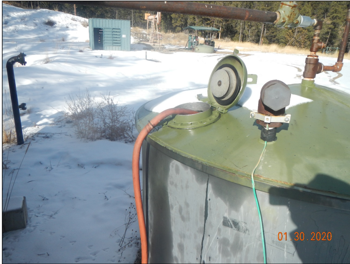
Photo 3. The lid is open on the tank. There are signs of spillage out of the tank.
