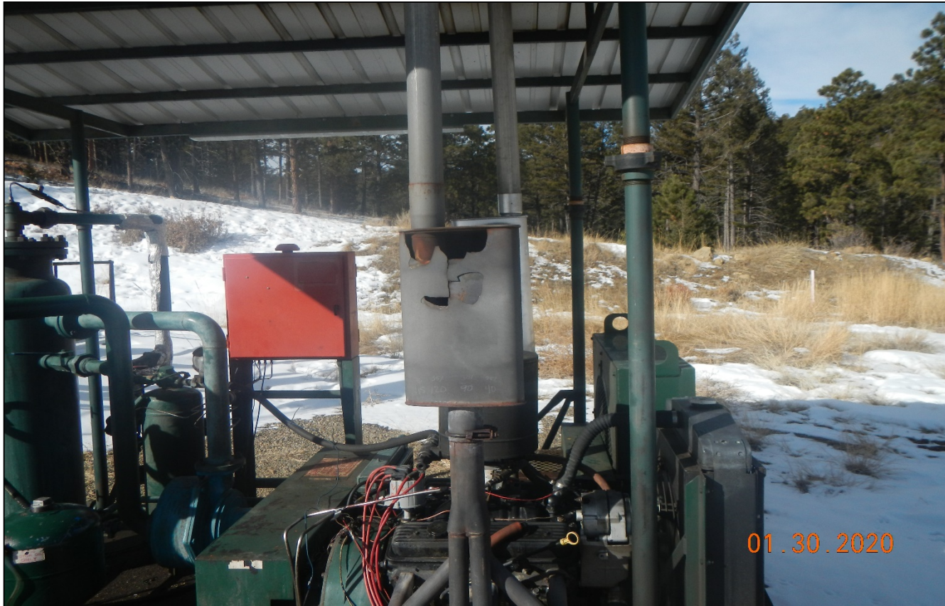
Photo 7. The muffler on the engine is broke apart causing the engine to be very loud. Needs to be maintained in good mechanical condition.
