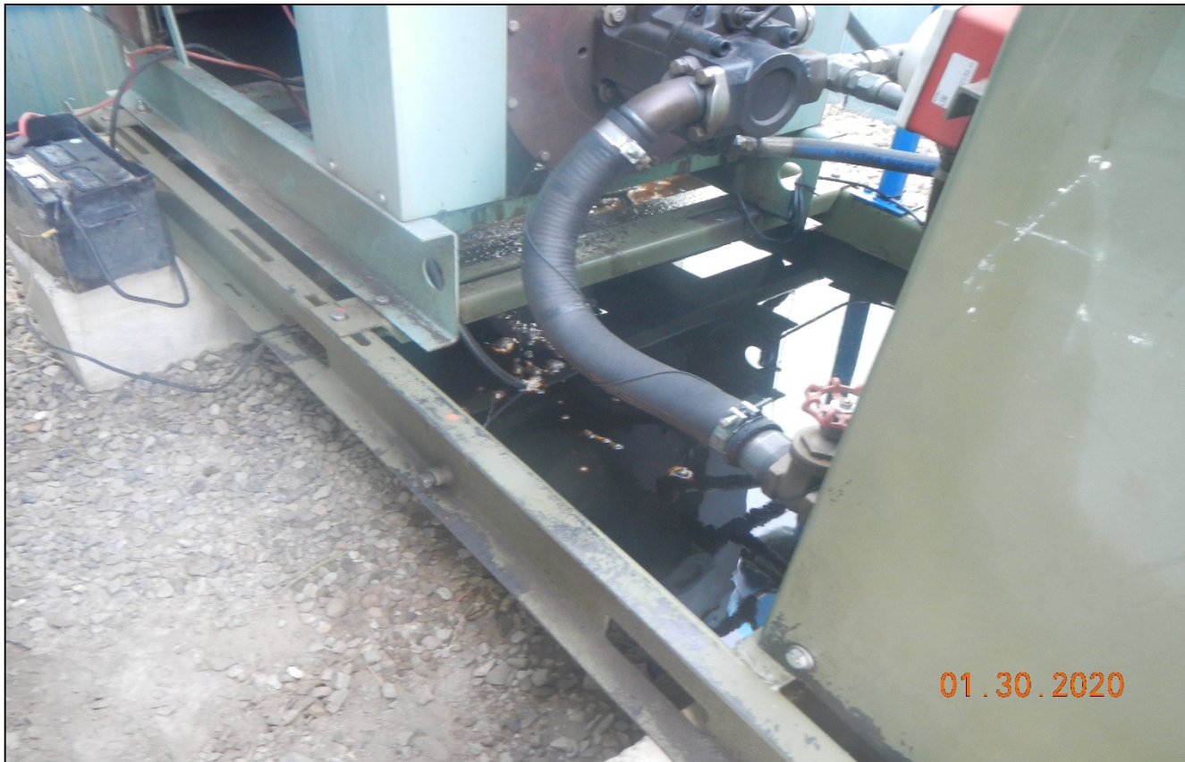
Photo 5. There is oily waste in the engine skid.
