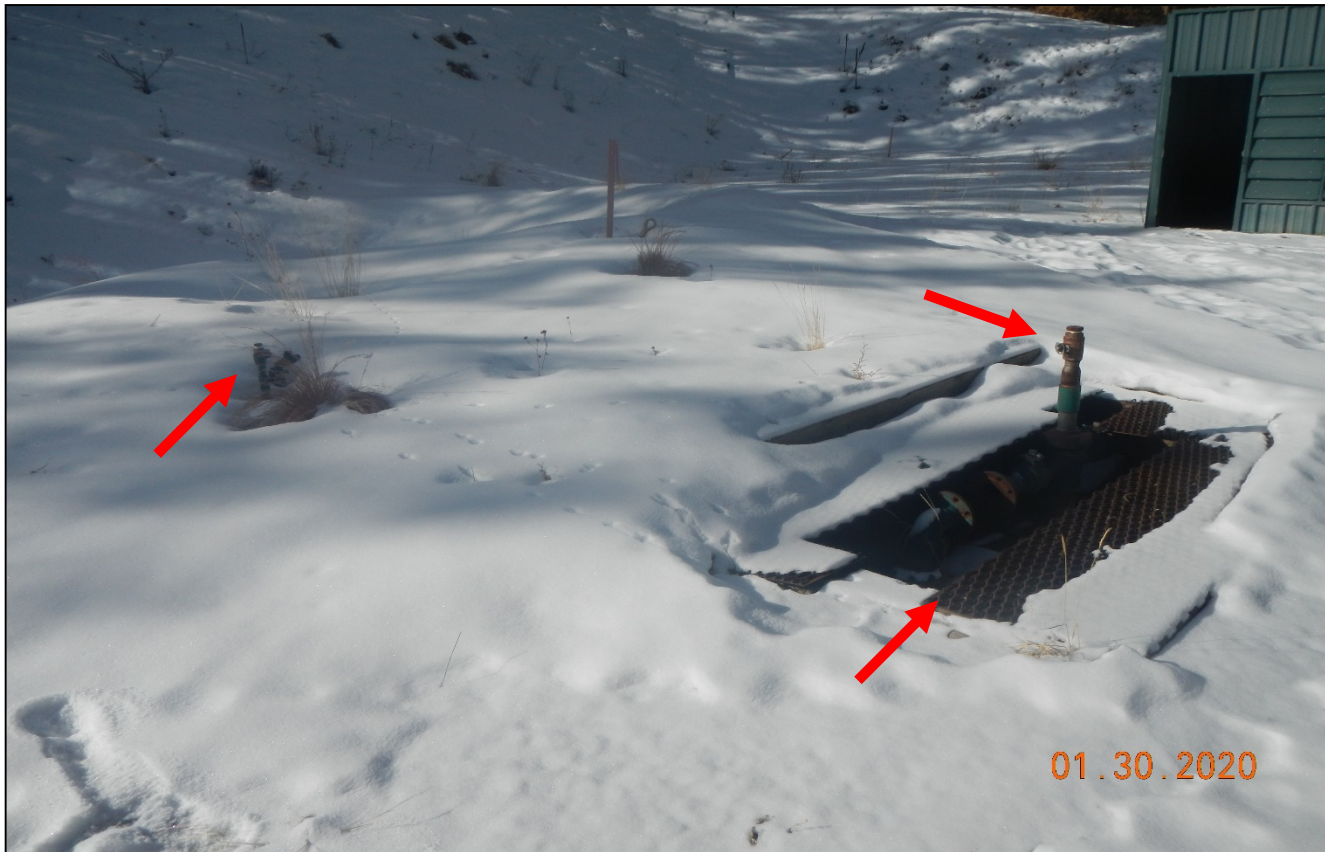
Photo 4. There is pipe riser with no LO/TO and clearly visible . The steel covers need to be placed to avoid entry.
