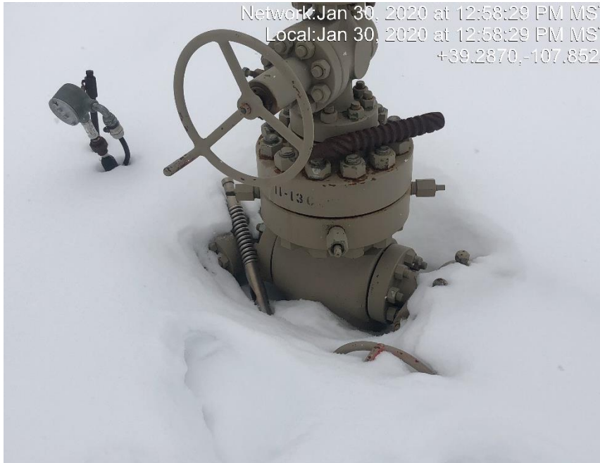
Photo #0501 Unused plunger and bumper spring.
