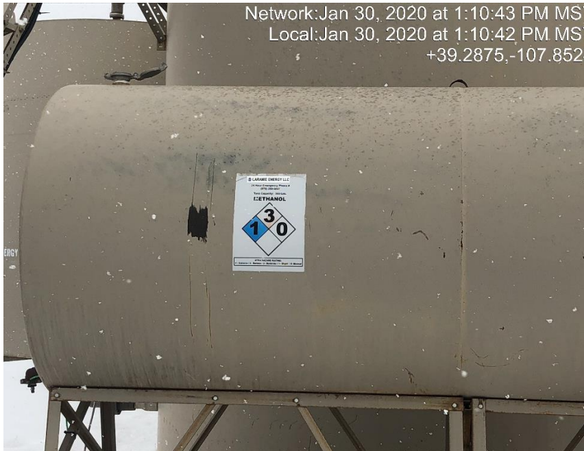
Photo #0502 1000 gallon methanol tank capacity inaccurate.
