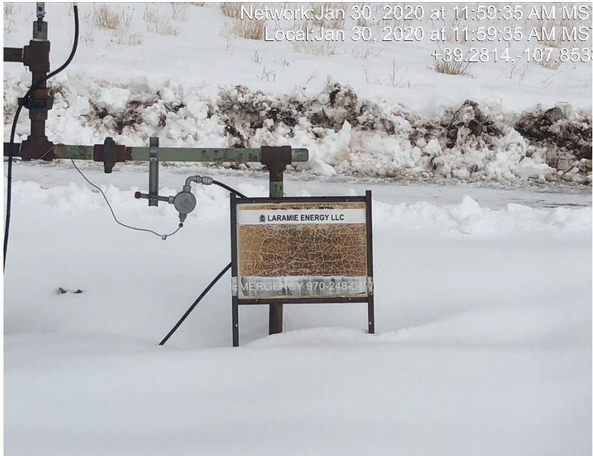
Photo #0495 Multiple wellhead signs weathered and not legible.
