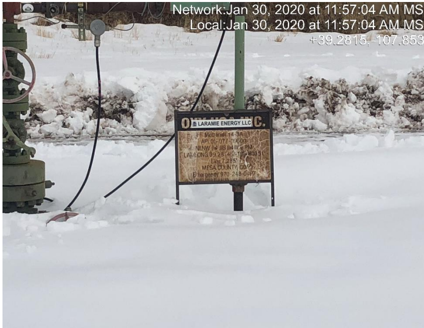
Photo #0493 Multiple wellhead signs weathered and not legible.
