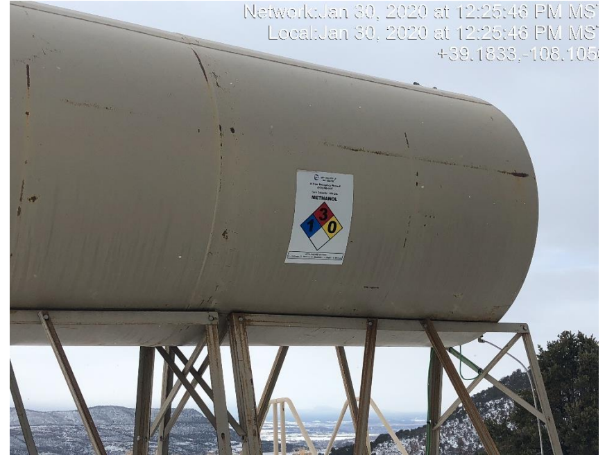
Photo #0497 1000 gallon methanol tank capacity label inaccurate.
