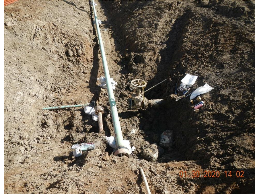
Work progressing to reportedly abandon flow lines within trench.
