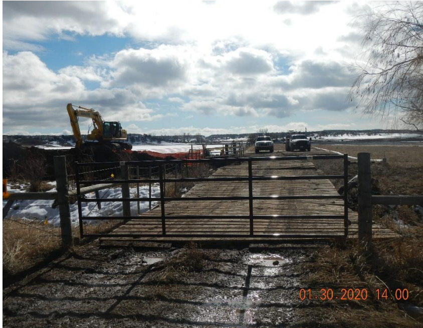
Matting over bridge for equipment to access release point.
