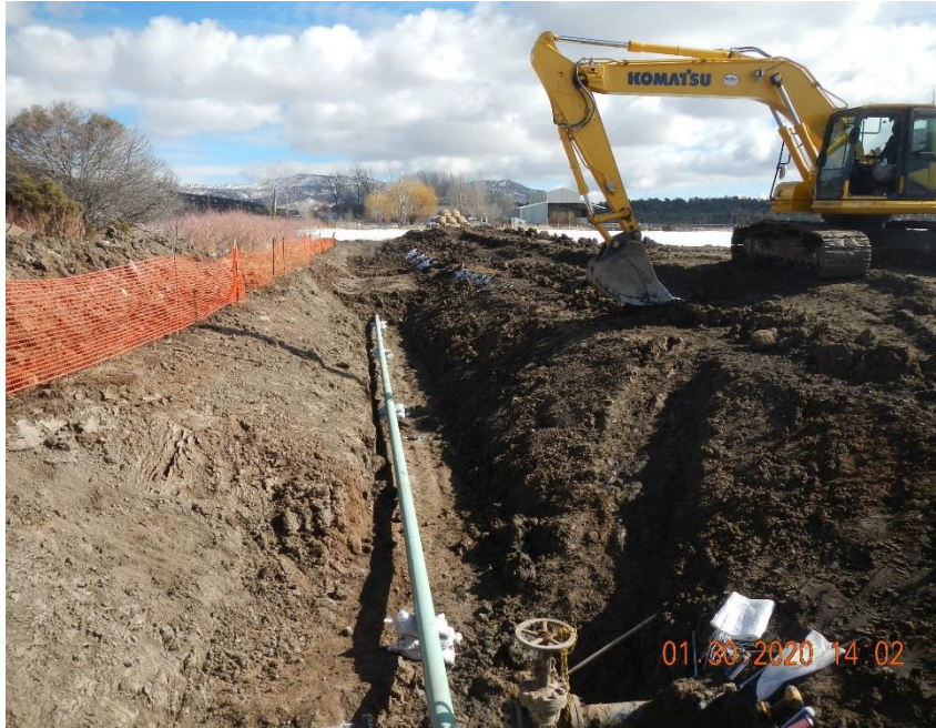
Replaced section of pipeline where release occurred.
