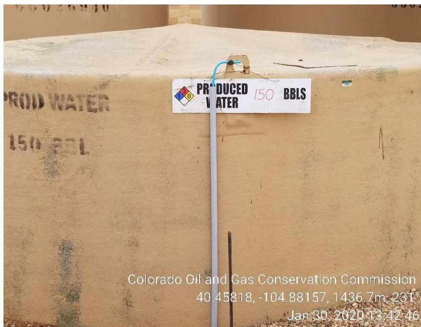
Photo 3: NFPA placard installed
