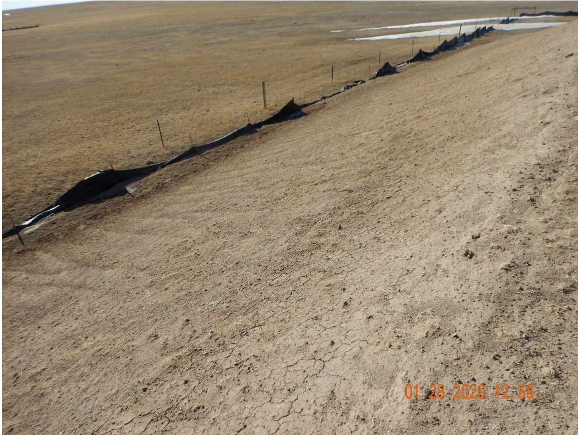
Photo 2. Photo taken from the topsoil stockpile, facing West. Photo illustrates topsoil has not been properly stabilized. Equipment tracking is only a temporary stabilization BMP.
