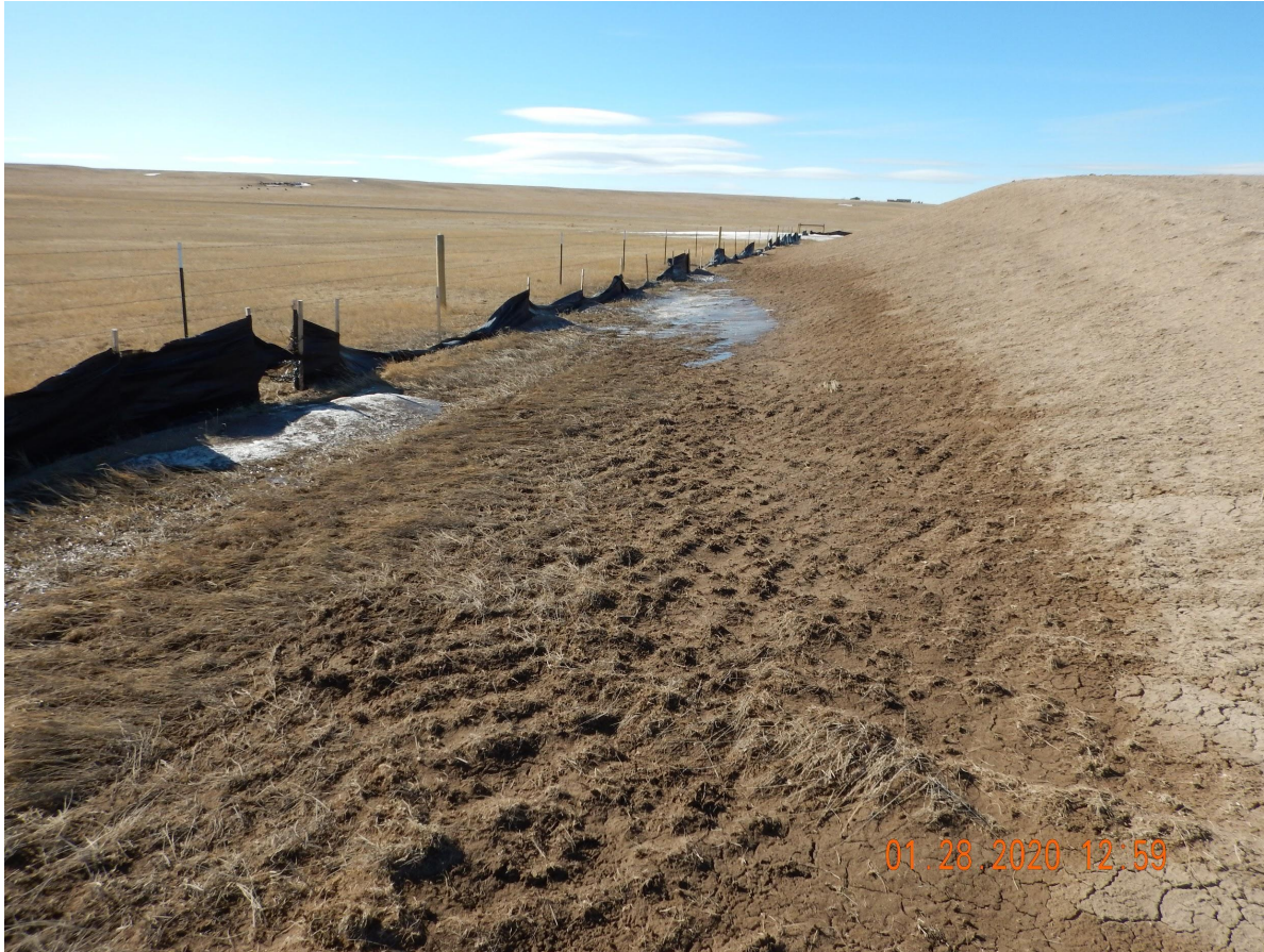
Photo 1. Photo taken from the topsoil stockpile, facing West. Photo illustrates stormwater BMP (silt fence) around the topsoil is not in proper functioning condition.
