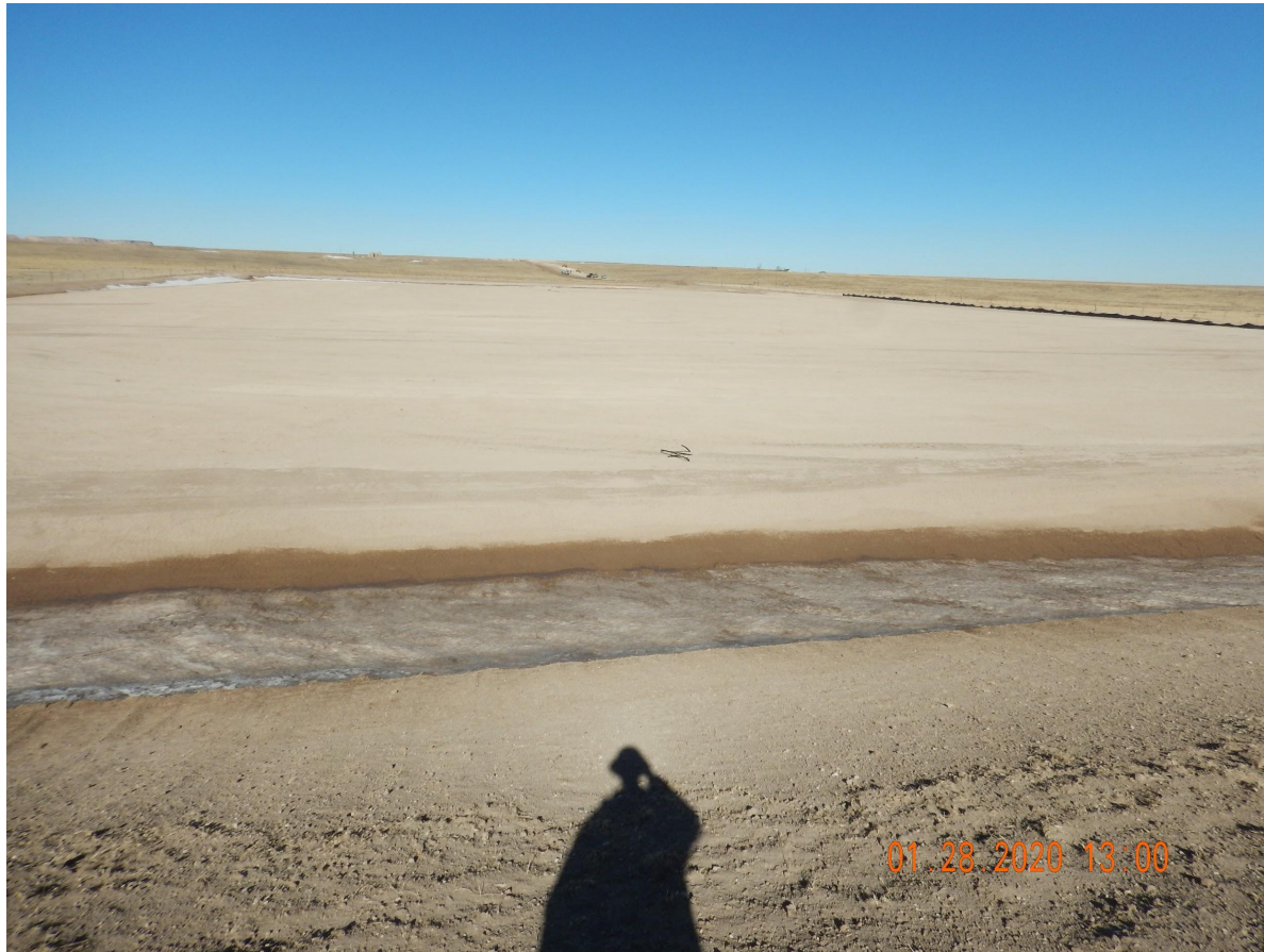
Photo 3. Photo taken from the topsoil stockpile, facing North. Photo illustrates Operator has not spud the location yet. Also, there is a retention around the entire well pad for stormwater management.
