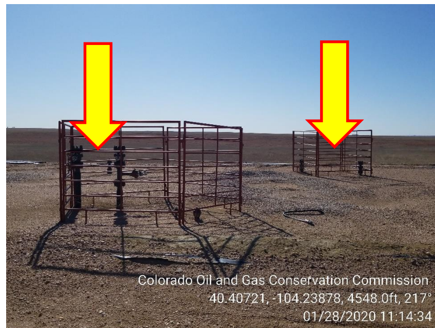
Photo 4 – Unmarked Risers between Separator and Compressor
