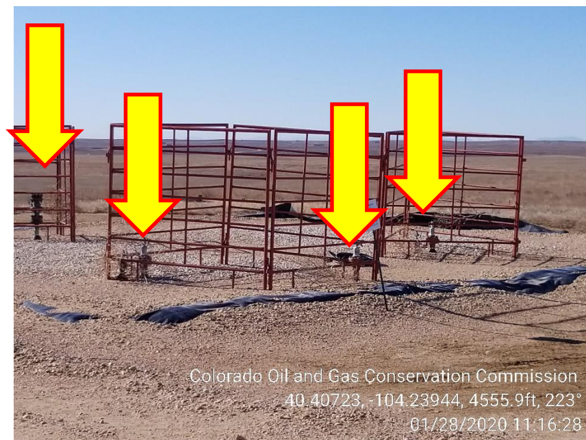
Photo 6 – Unmarked Risers in Southwest Corner of location
