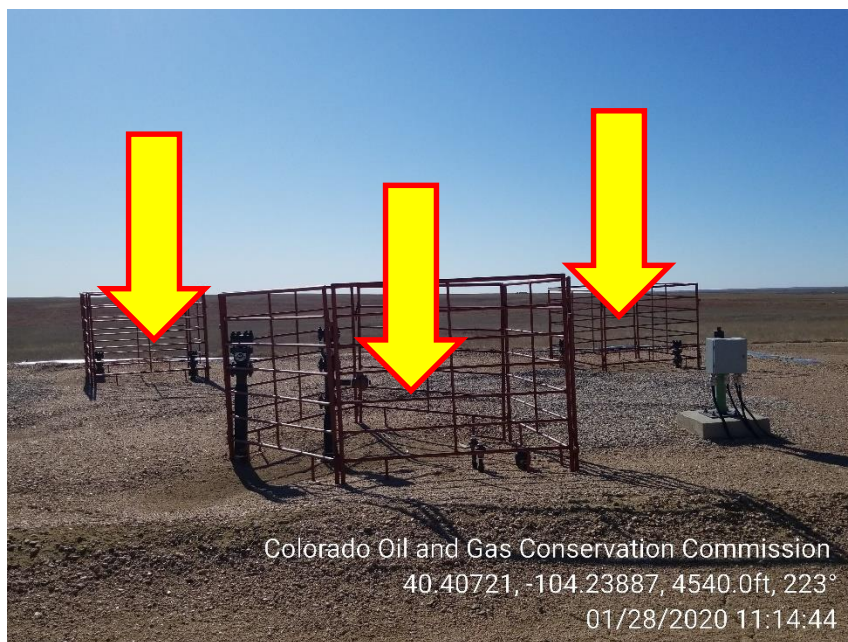
Photo 5 – Unmarked Risers between Separator and Compressor
