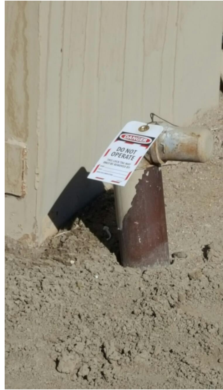
Figure #5 Risers have been tagged.
