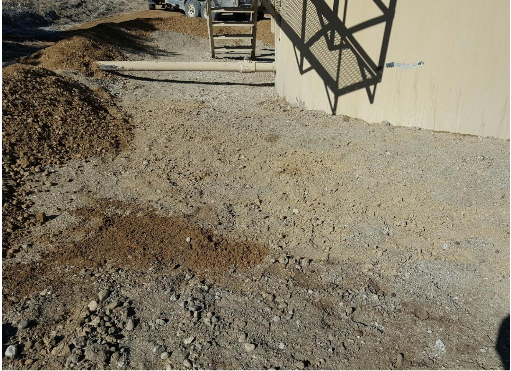
Figure #1 Stained soil has been removed. Leak has been fixed.
