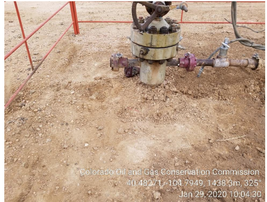
Photo 6: Stained soil removed
