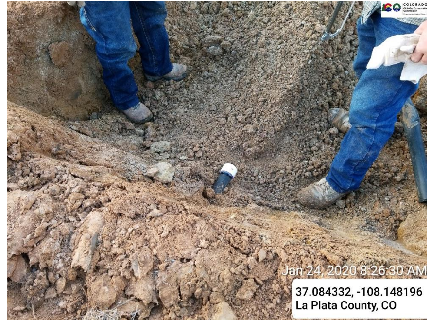
PVC flowline cut and capped.
