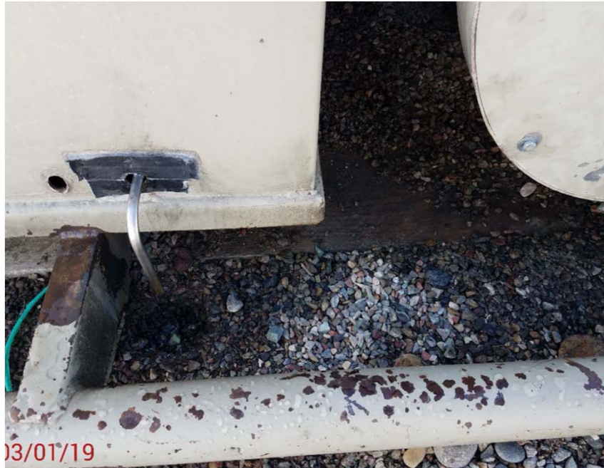
Staining around separators from previous inspection
