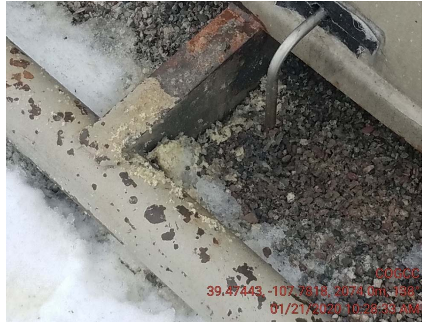
Staining around separators
