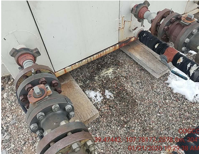
Staining around separators
