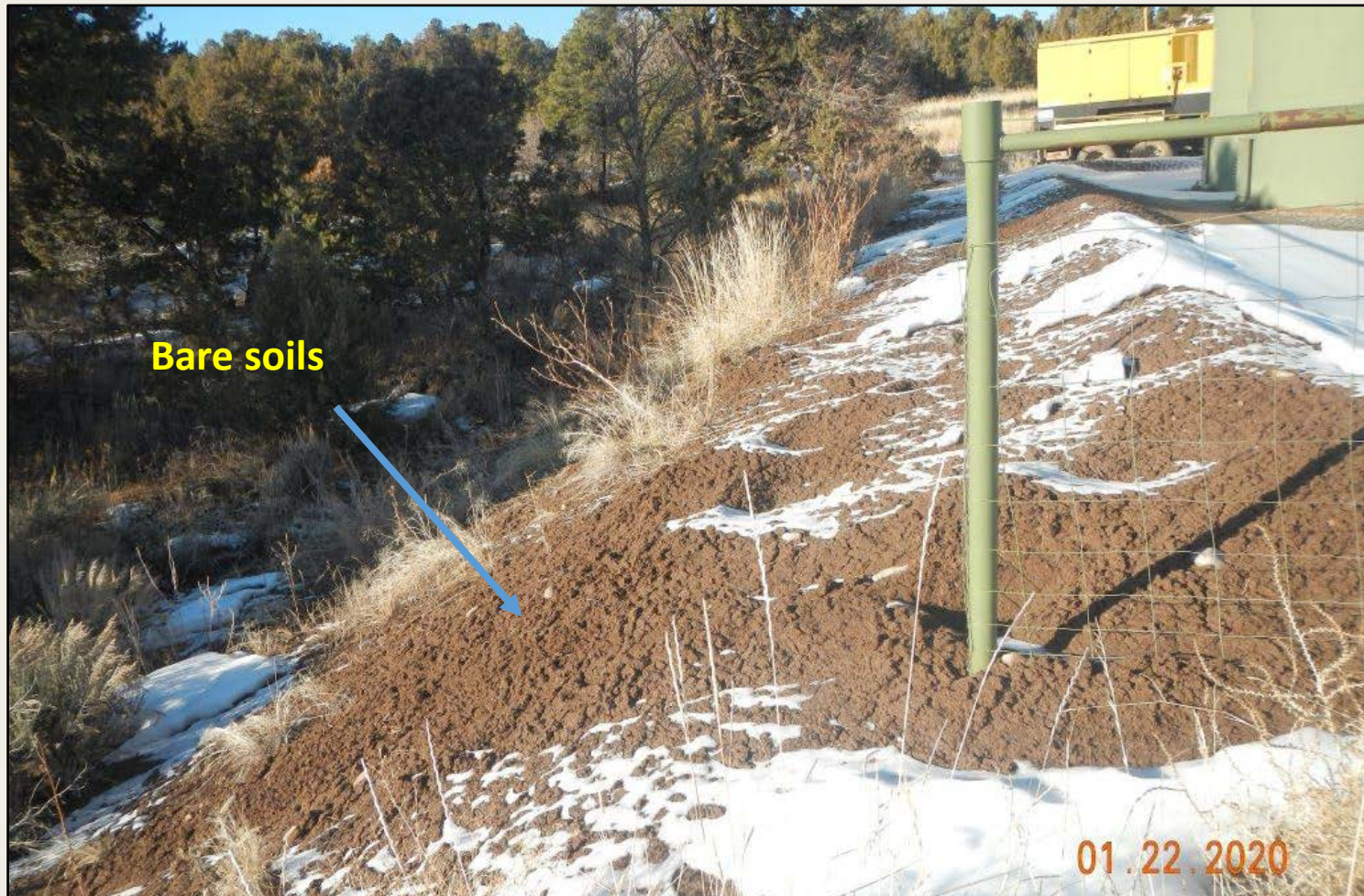
Photo 7. View of bare soils within the southwestern project area. Erosion controls are needed to stabilize bare soils here.
