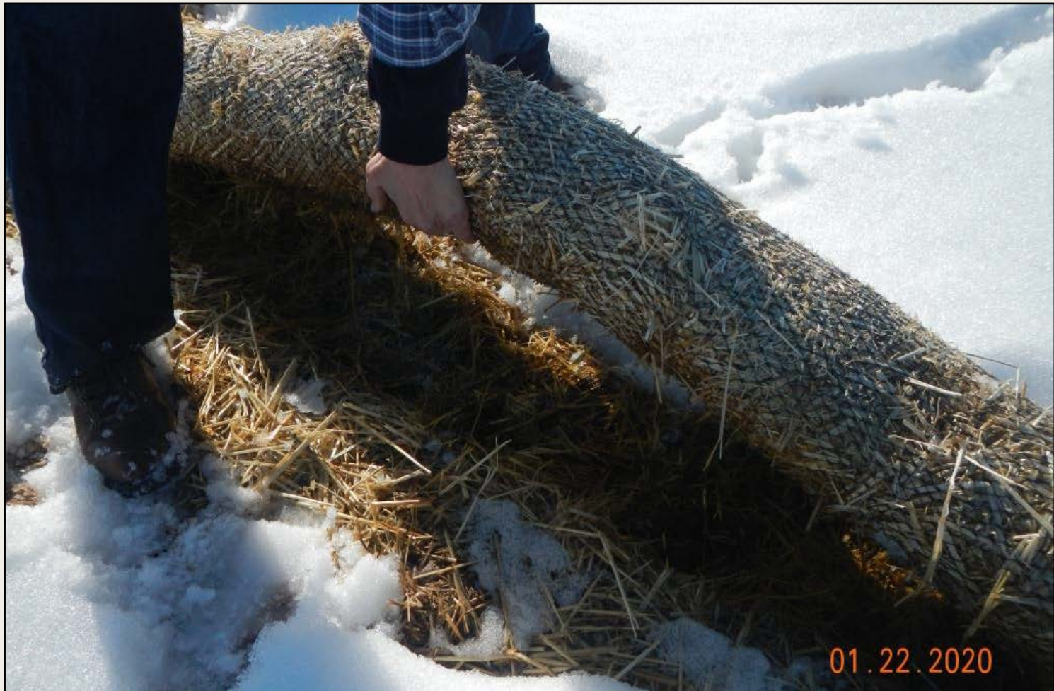
Photo 4. View of area beneath wattle that shows that wattle is not properly trenched within the soil.
