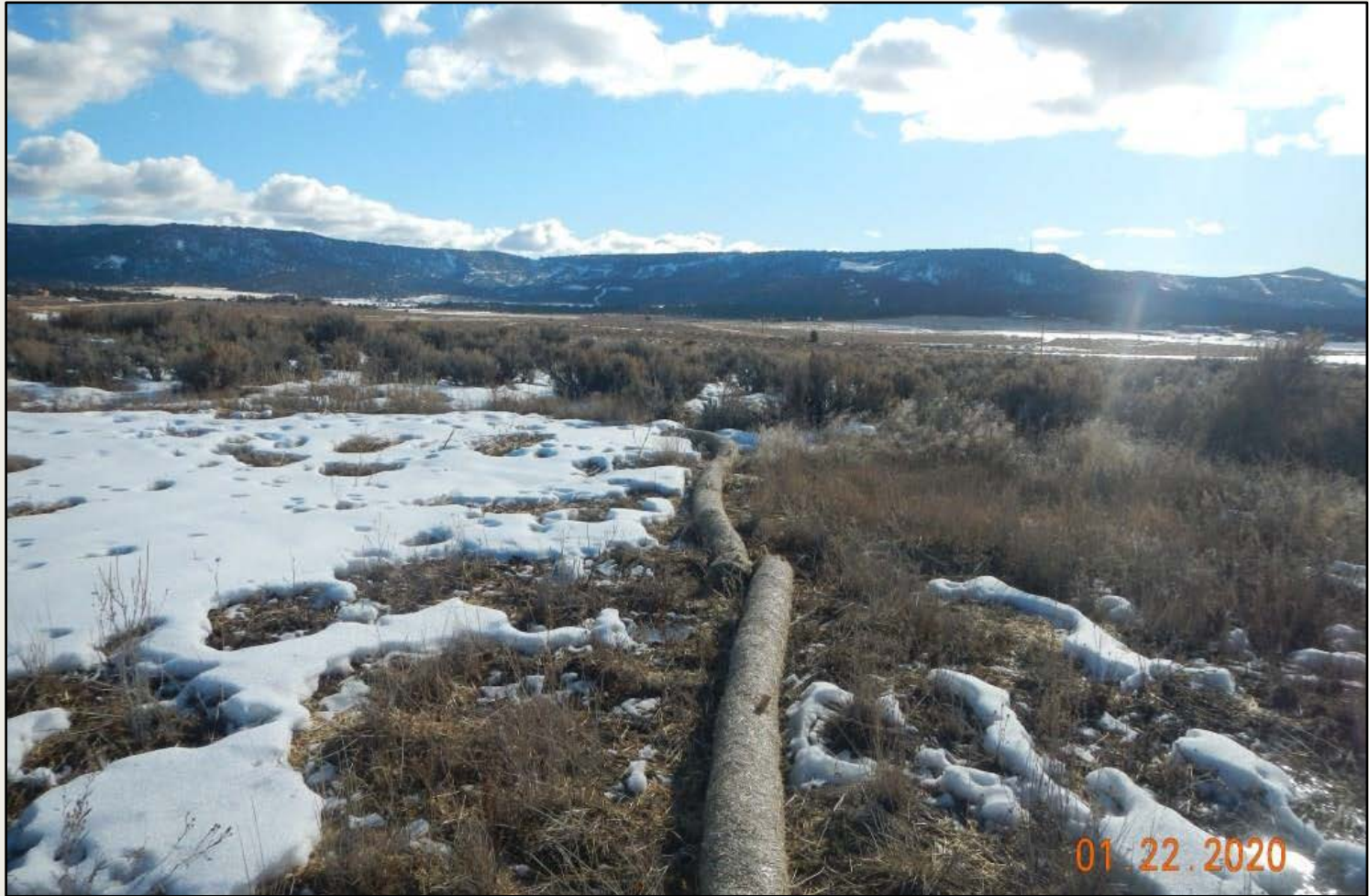
Photo 2. View of wattles placed along the western edge of the project area.
