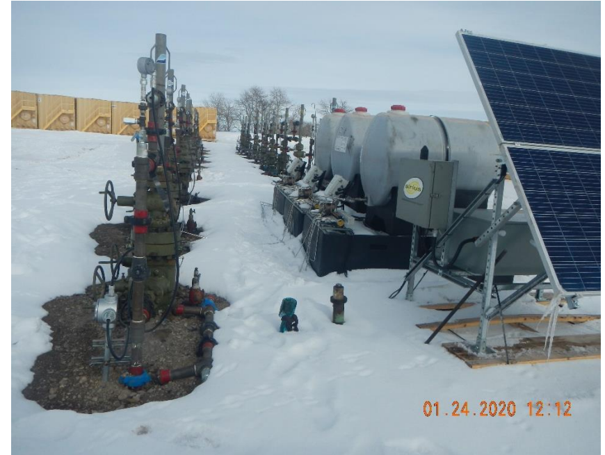
2 risers at wells are unused and not capped.
