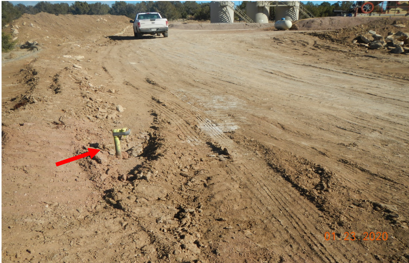
Photo 6. There is a pipe riser at west side that is not clearly visible or protected.
