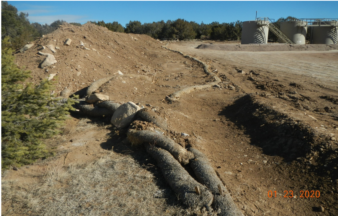
Photo 7. Wattle are displaced in areas around the location. BMP's must be maintained at all times.
