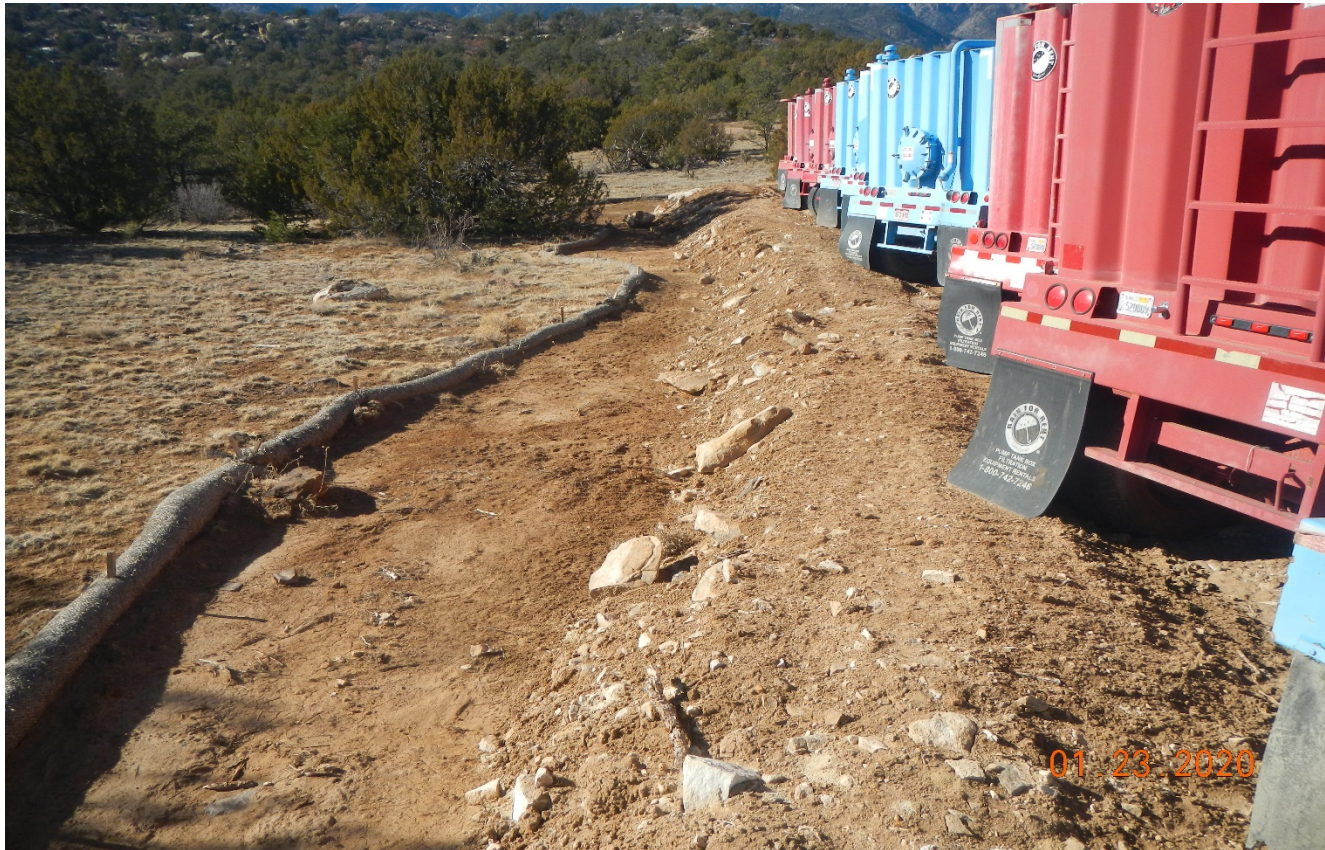
Photo 15. There are wattles installed around the southeast perimeter however stormwater will run down hill along the wattles.
