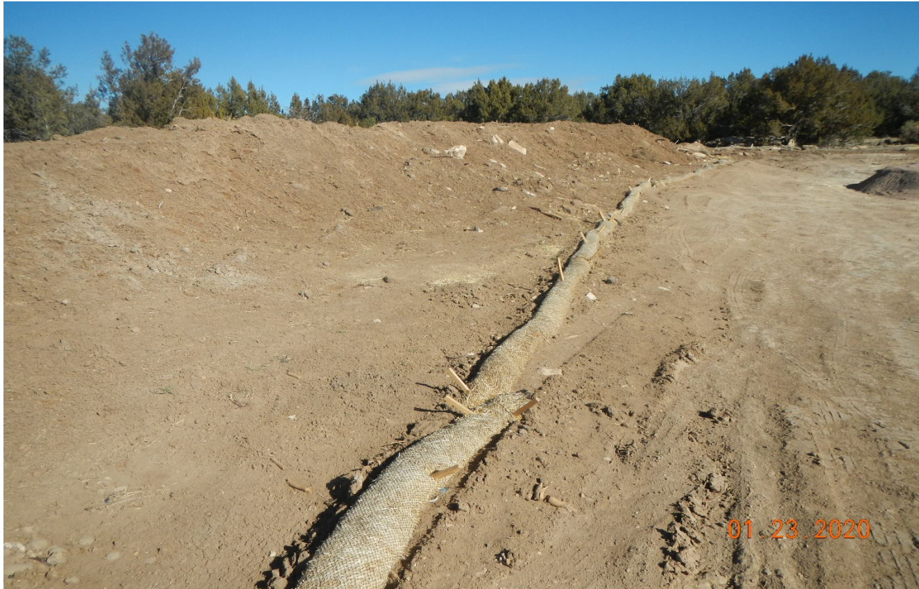
Photo 8. Topsoil pile at west side of the location. The topsoil pile is not stabilized and protected. A portion of the topsoil will need to be used for interim reclamation. The remaining portion must be seeded and stabilized.
