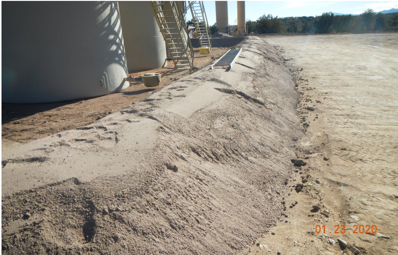
Photo 10. The berms around the tank battery are not compacted.
