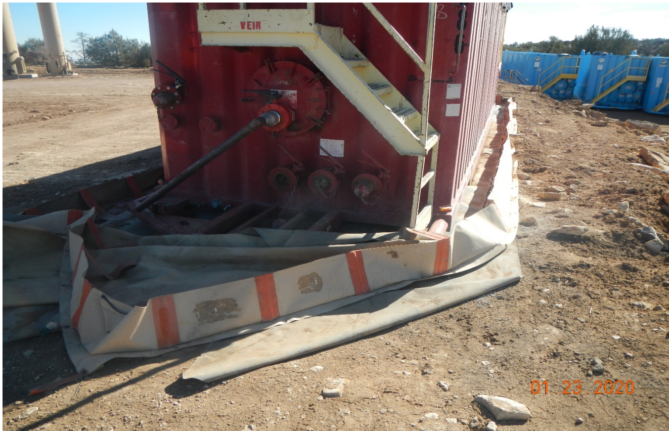
Photo 11. The secondary containment around the tank is not adequate to contain spill.
