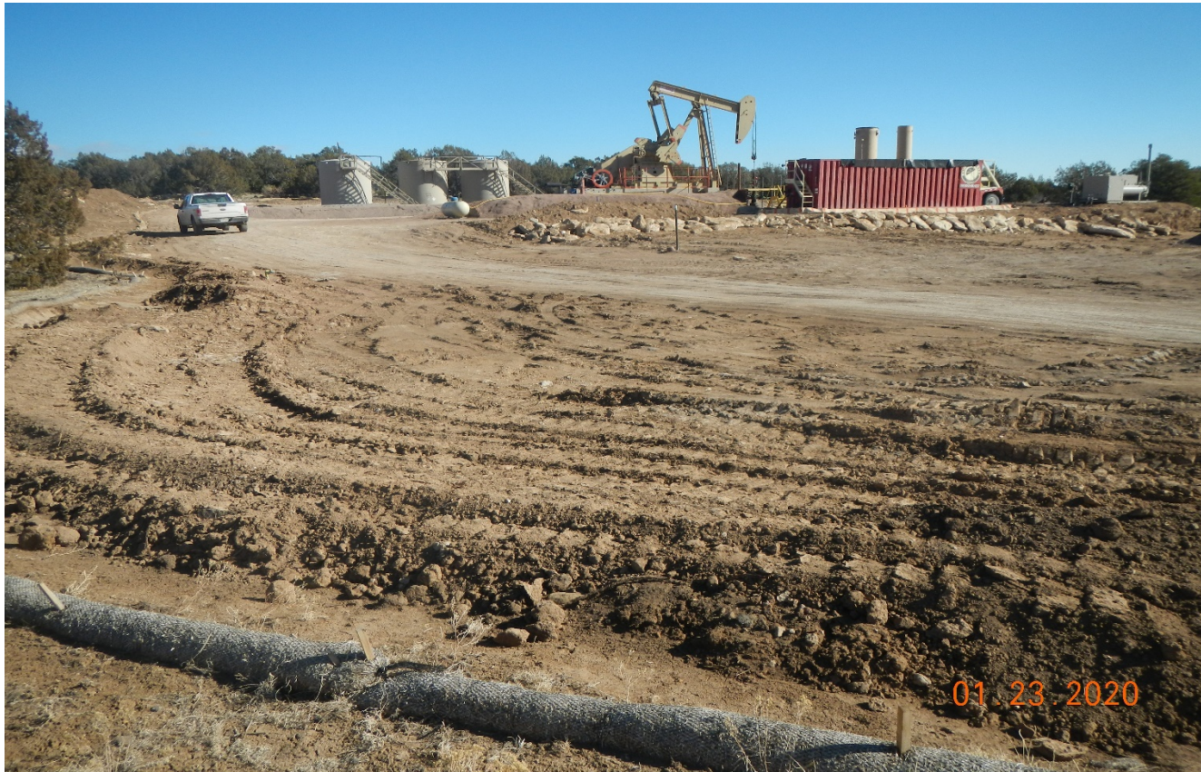
Photo 5. West side of the location facing northeast. Unused areas of the location must be reclaimed. Disturbed soils are susceptible to erosion.
