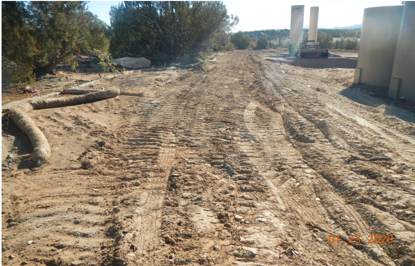
Photo 9. North side of the location facing east. The wattles are displaced and disturbed soils are not stabilized.
