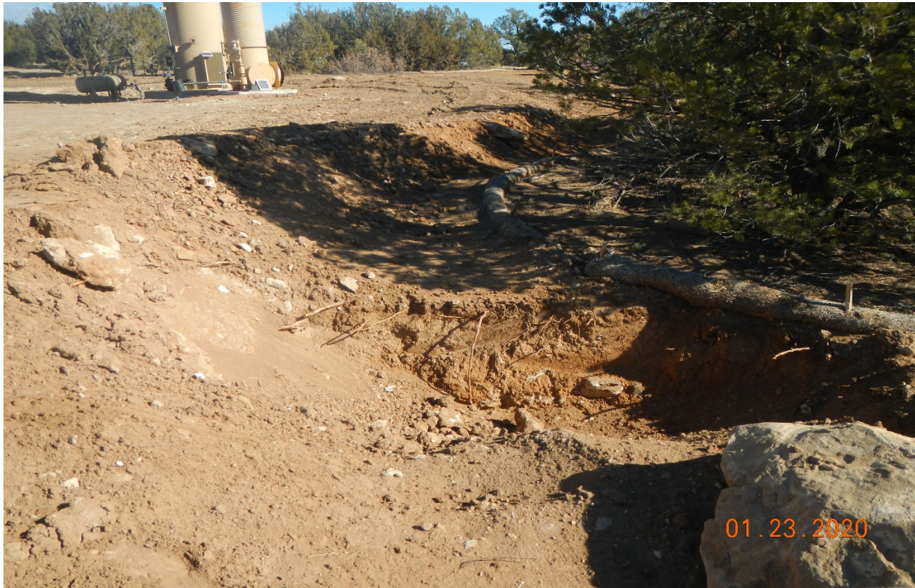
Photo 14. There is a hole at the east side of location which may be an incomplete sediment trap. BMP's must be implemented in accordance with good engineering practice and must be maintained at all times.
