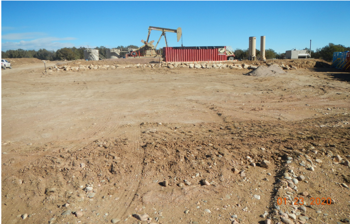
Photo 4. Facing north toward the location. Interim reclamation has not been performed. Unused areas must be reclaimed.
