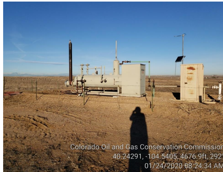
Photo #2 Separator & Meter Run
