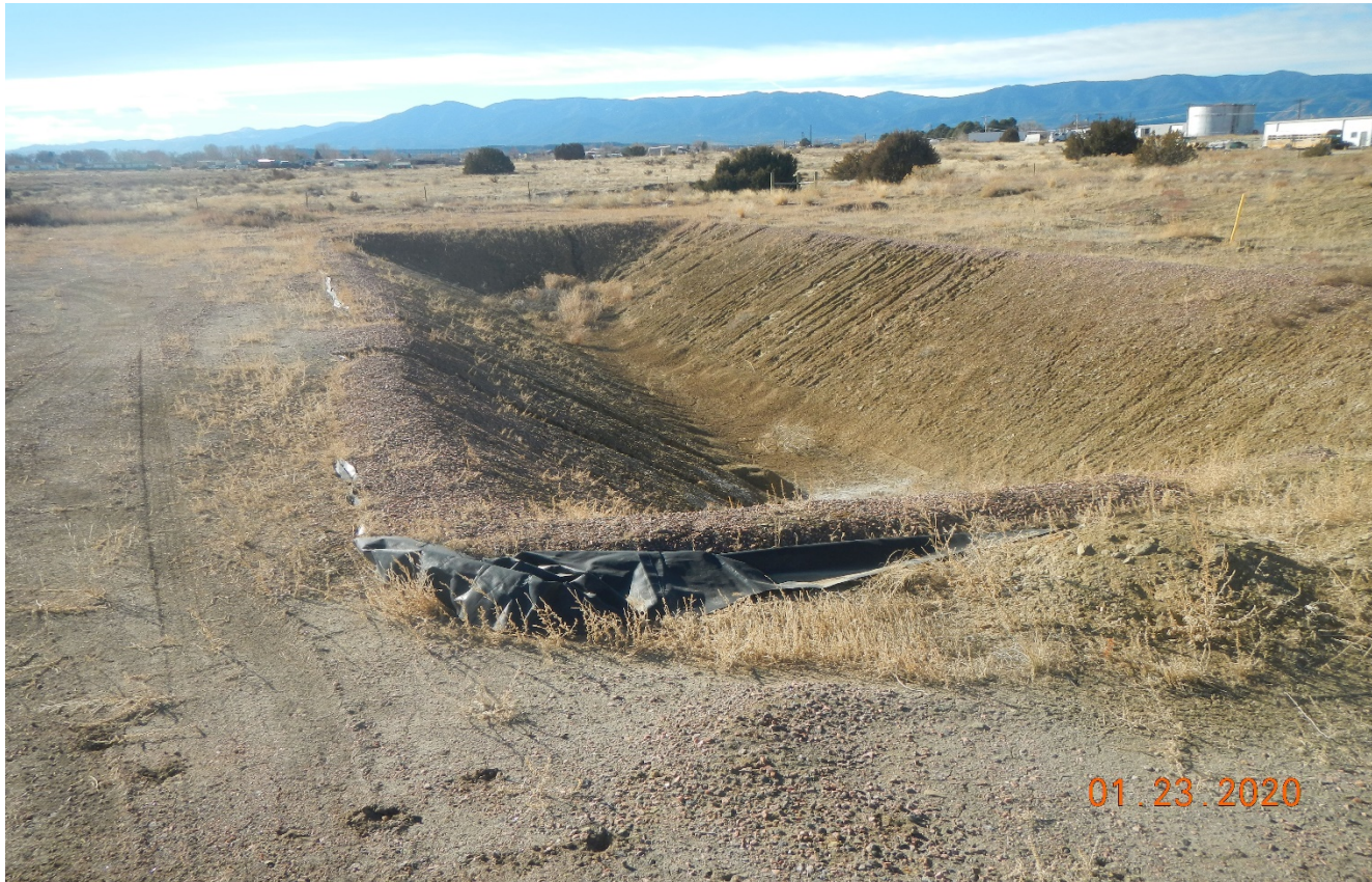
Photo 4. The drilling pit has not been closed and reclaimed as required.
