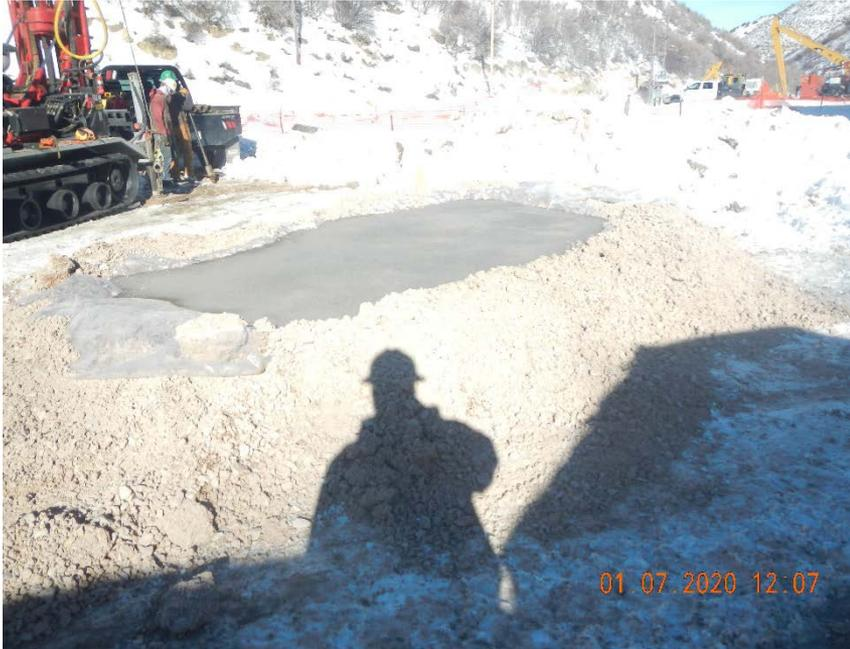
Photo #2 Containment area has material that was hydro-excavated from the top 3-4 feet. There was no observable impact (olfactory or visual) in the holes that were hydrovaced. Weather was below freezing. Wesco should remove fluid and solids as soon as possible.
