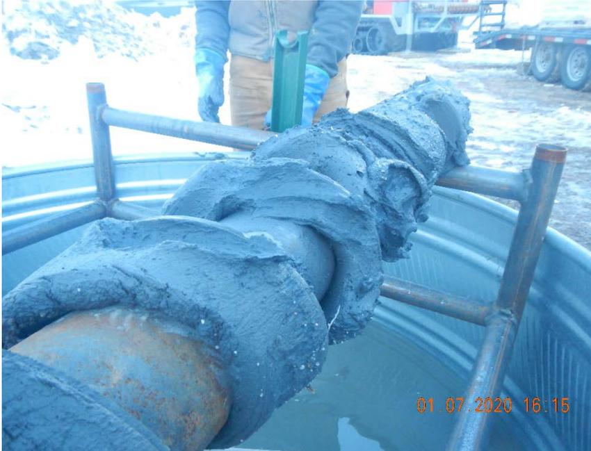
Photo #25 Cleaning of auger bit. Note: kiddie pool catchment basin.
