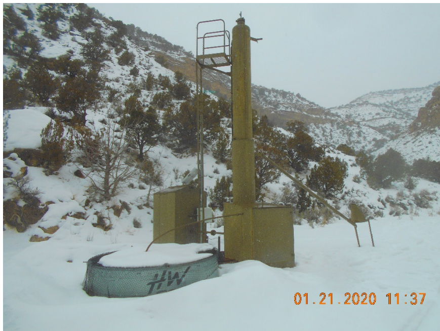
Meter housing, Dehydrator with blowdown tank
