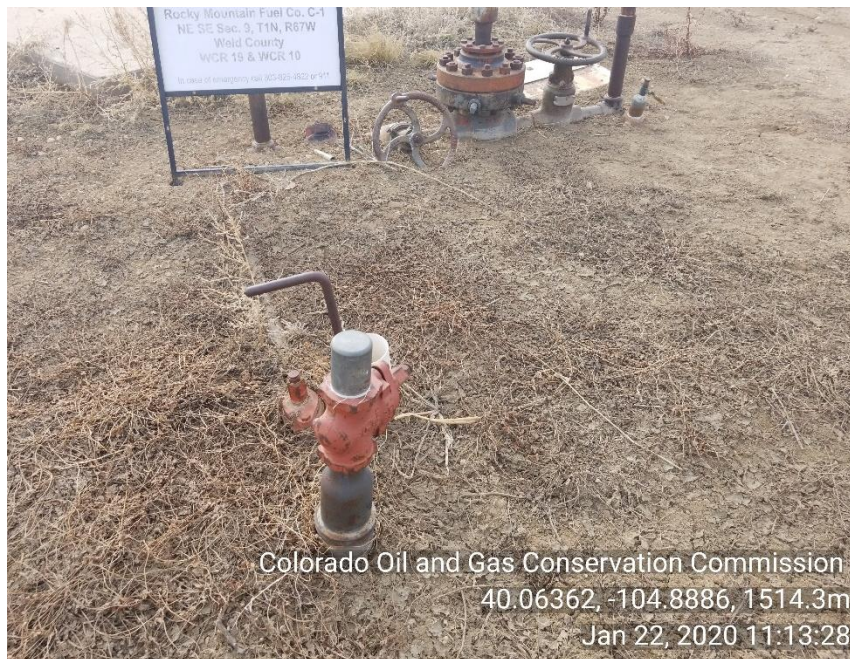
Photo 7 Unmarked unused riser not LOTO
