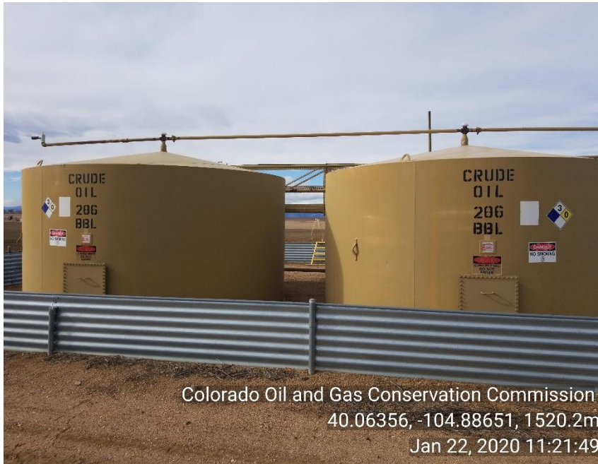
Photo 15 NFPA placards faded need to be replaced.
