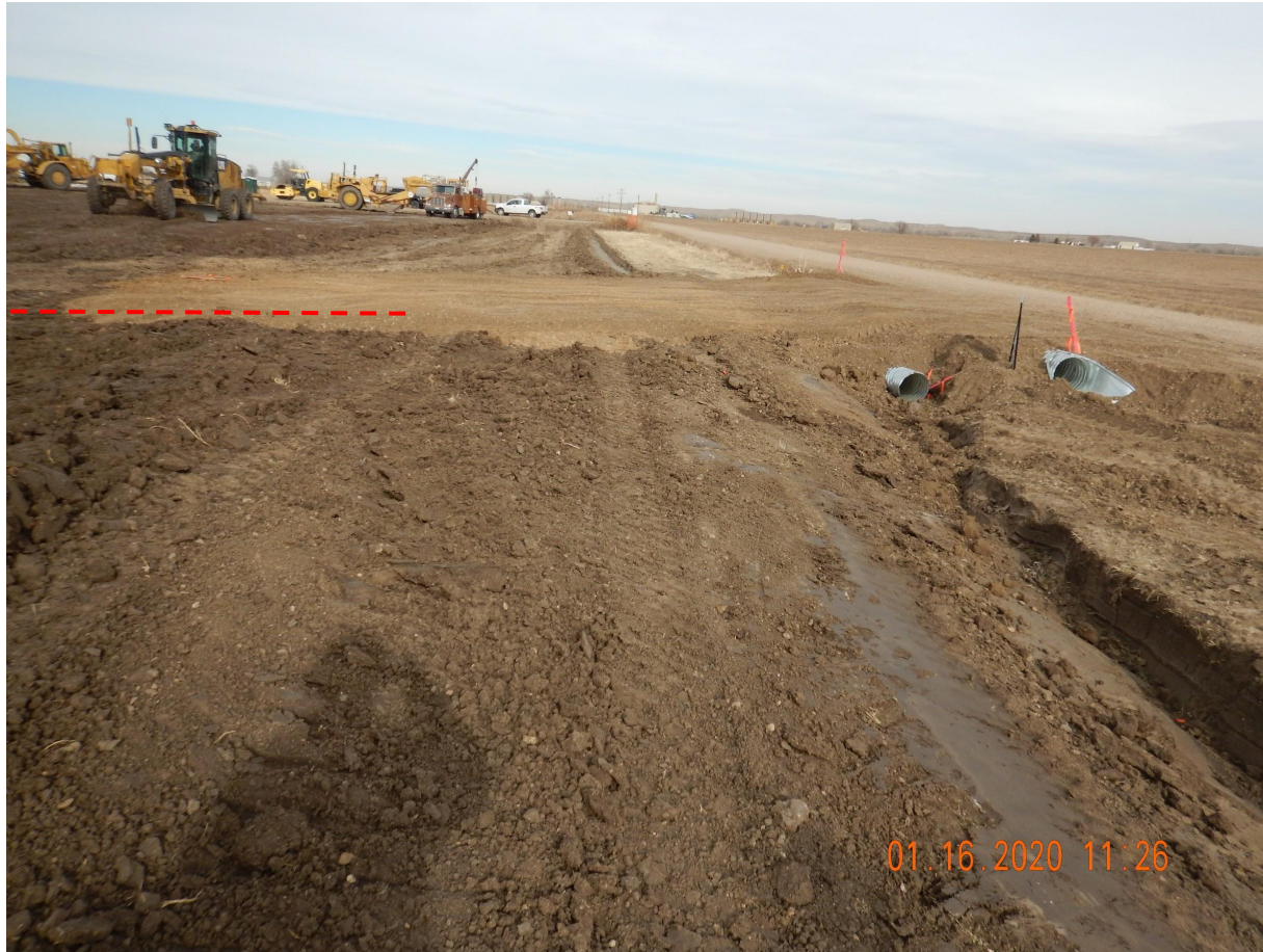
Photo 2. Photo taken from the eastern perimeter of location, facing North. Photo illustrates a ditch BMP which is directed to a sediment trap (still in-process) along with culverts.
