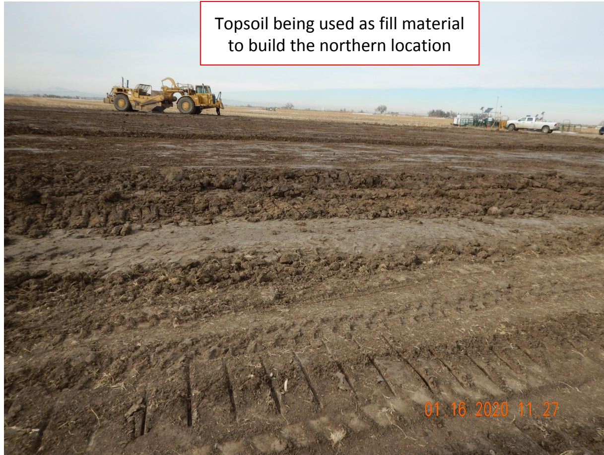
Photo 3. Photo taken from the eastern perimeter of location, facing West. Photo illustrates topsoil being used as fill material to build up the northern part of the location.
