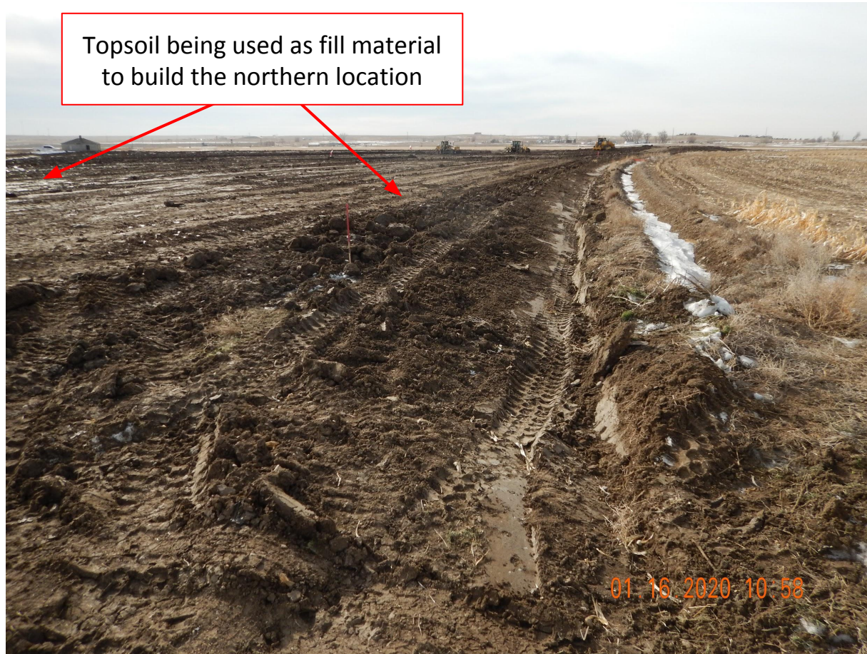
Photo 1. Photo taken from the northwestern perimeter of location, facing South. Photo illustrates a ditch BMP which is directed to a sediment trap (still in-process).
