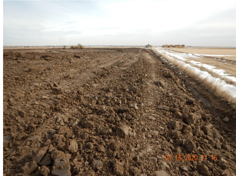
Photo 7. Photo taken from the southern perimeter of location, facing East. Photo illustrates topsoil being stored along the southern perimeter of location.
