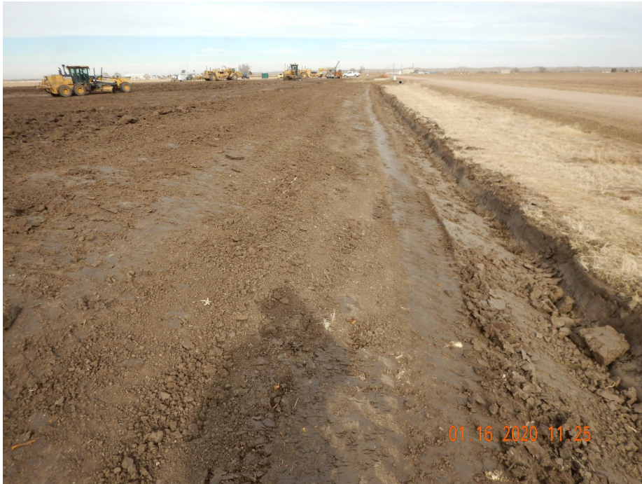
Photo 8. Photo taken from the southeastern perimeter of location, facing North. Photo illustrates topsoil being stored along a portion of the eastern perimeter of location. See comments under Photo 1 regarding the ditch BMP.
