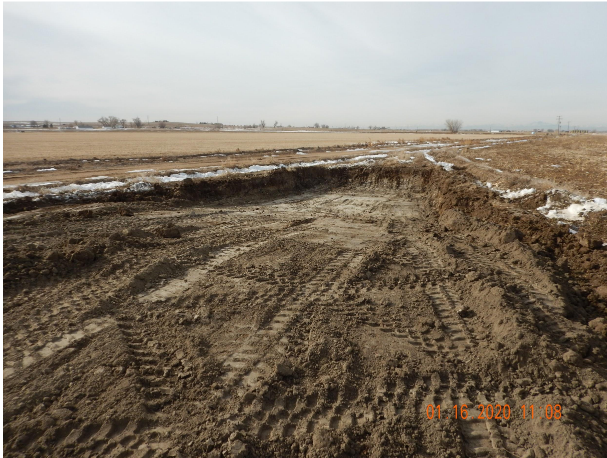
Photo 5. Photo taken from the southwestern perimeter of location, facing Southwest. Photo illustrates the sediment trap which is still in-process of being constructed.
