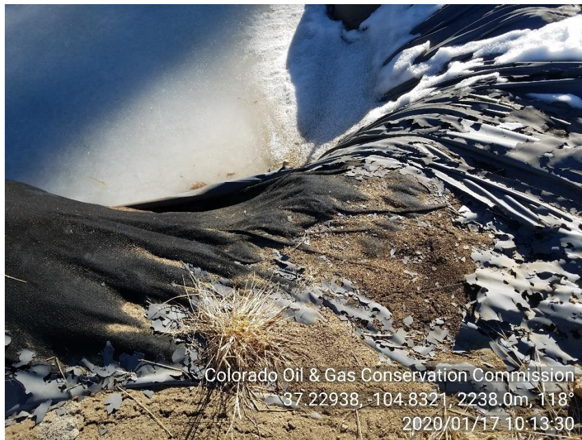
PHOTO 5: ANOTHER IMAGE OF PIT LINER DETERORATION.
