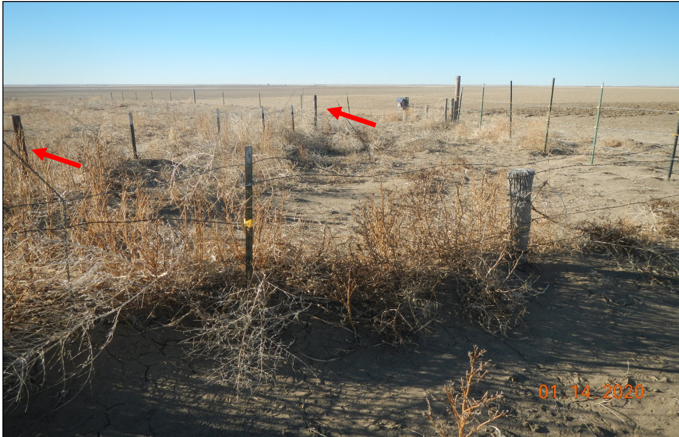
Photo 1. The area where the cattle existed is now fenced off. This area has accumulated sand and has filled in the cattle guard. Arrow points to the two cattle guard posts. The cattle guard will need to be removed and area reclaimed. Lat/Long: 38.86674/-102.66708
