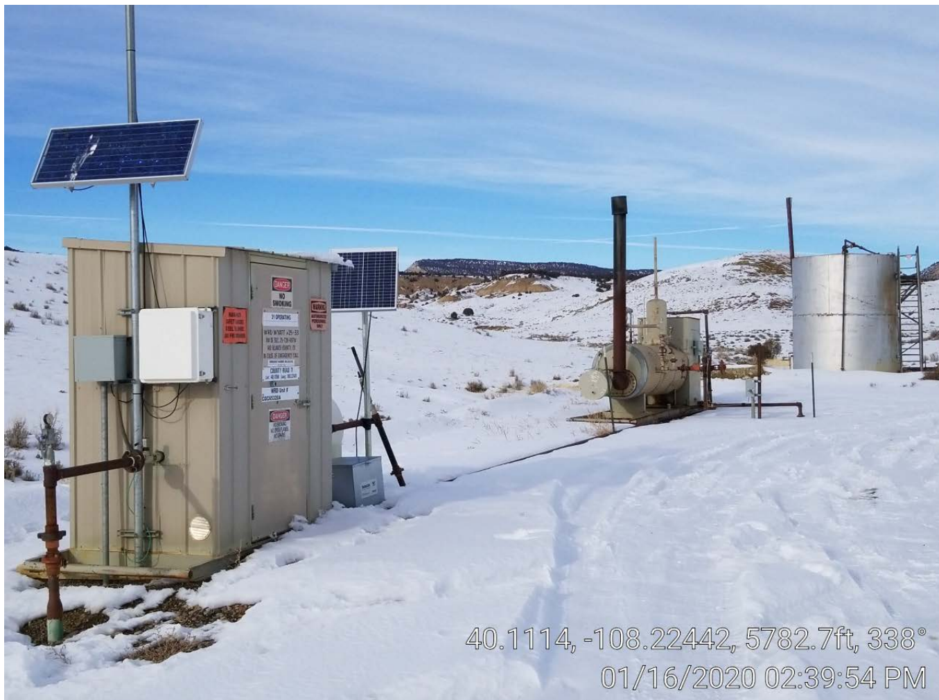
Photo 3. Meter building, separator, and tanks.
