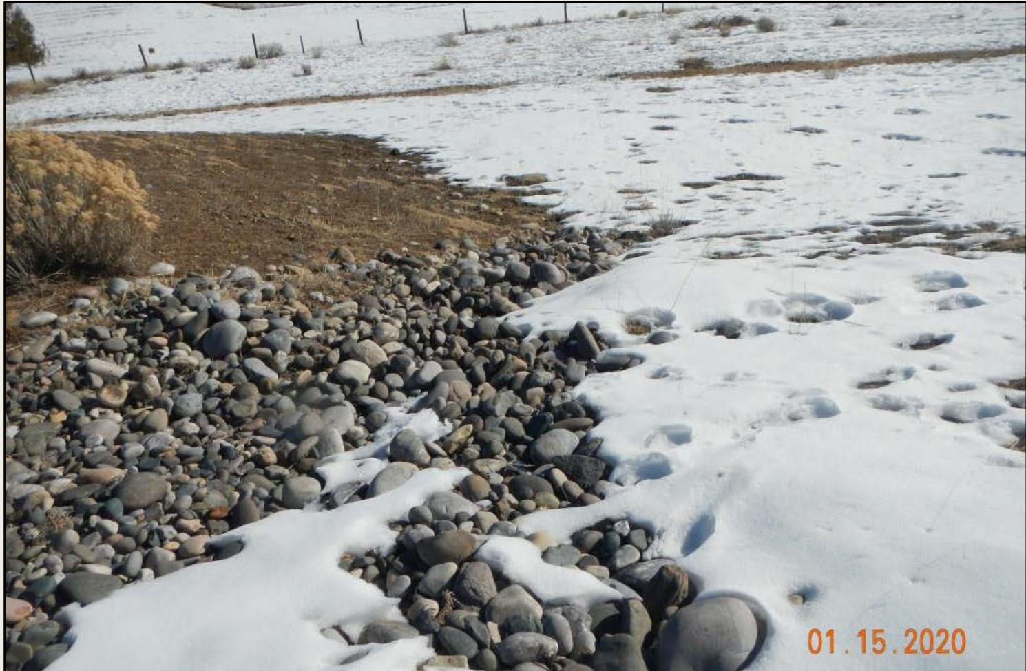
Photo 3. View of cobble within the southeastern project area, although functionality is not assessed due to snow cover. Operator should note that cobble rock is not considered a BMP, as it does not effectively reduce energy of stormwater flows. Course rock is needed where rock is used as a stormwater BMP. Operator needs to continue to monitor stormwater erosion and apply BMPs according to good engineering practices when/where stabilization is needed.
