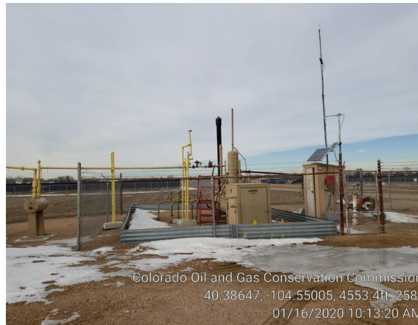
Photo #4 Separator & Meter Run
