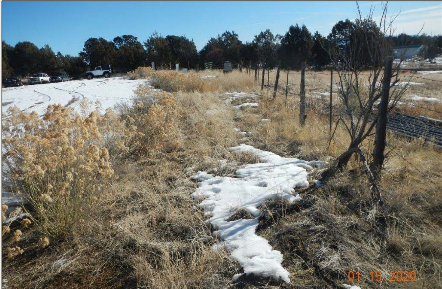
Photo 2. View of the southern fill slope from the southwestern corner facing eastward. Revegetation is progressing with grasses such as sand drop seed and western wheatgrass. Jointed goatgrass, an annual grass species identified in 2018 inspection needs treatment in spring (before flowering) if present.
