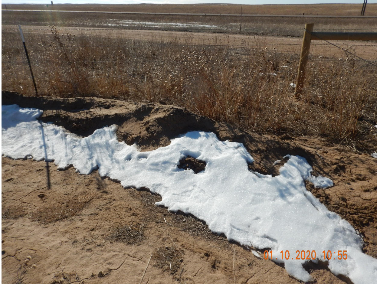
Photo 6. Photo taken from the southwestern perimeter of the location, facing South. Photo illustrates an insufficient ditch BMP installed.
