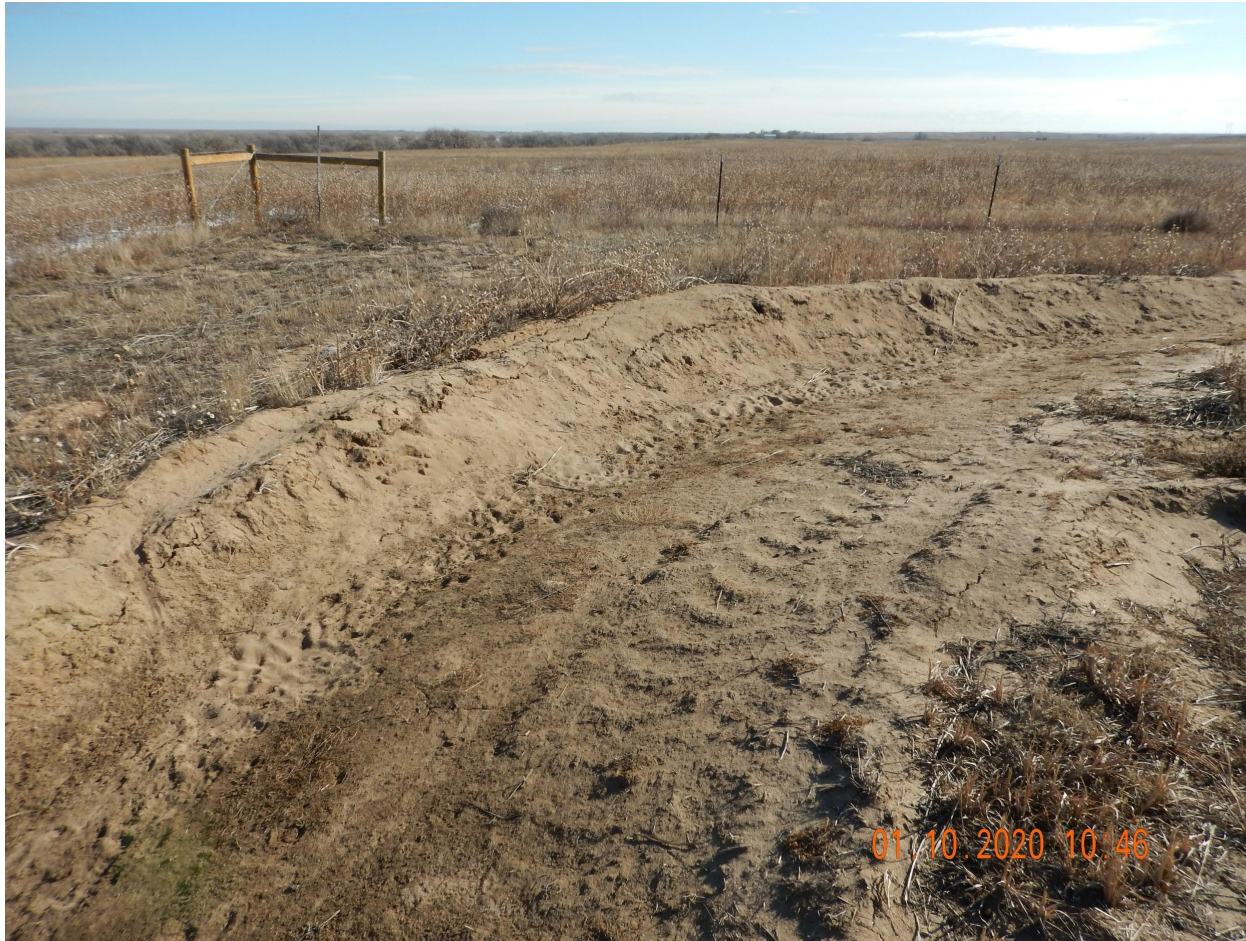
Photo 4. Photo taken from the northeastern perimeter of location, facing East. Photo illustrates there is no stabilized outlet, only a ditch BMP. Although there was no observed discharge from location, a ditch by itself is not sufficient.
