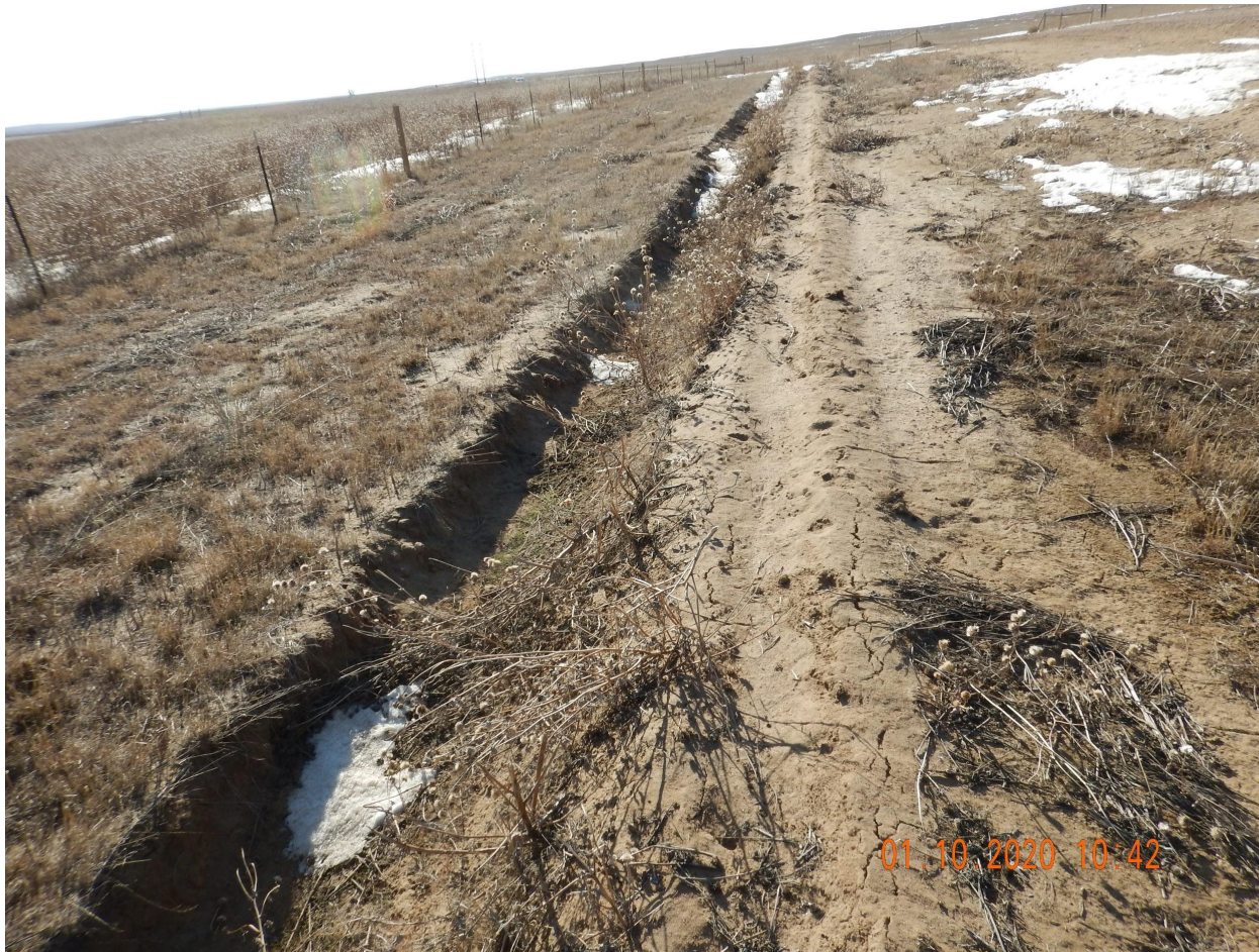
Photo 3. Photo taken from the eastern perimeter of the location, facing South. Photo illustrates a ditch BMP. Although there was no observed discharge from location, the ditch BMP has not been constructed in accordance with good engineering practices (i.e., proper depth and 2:1 side slopes).
