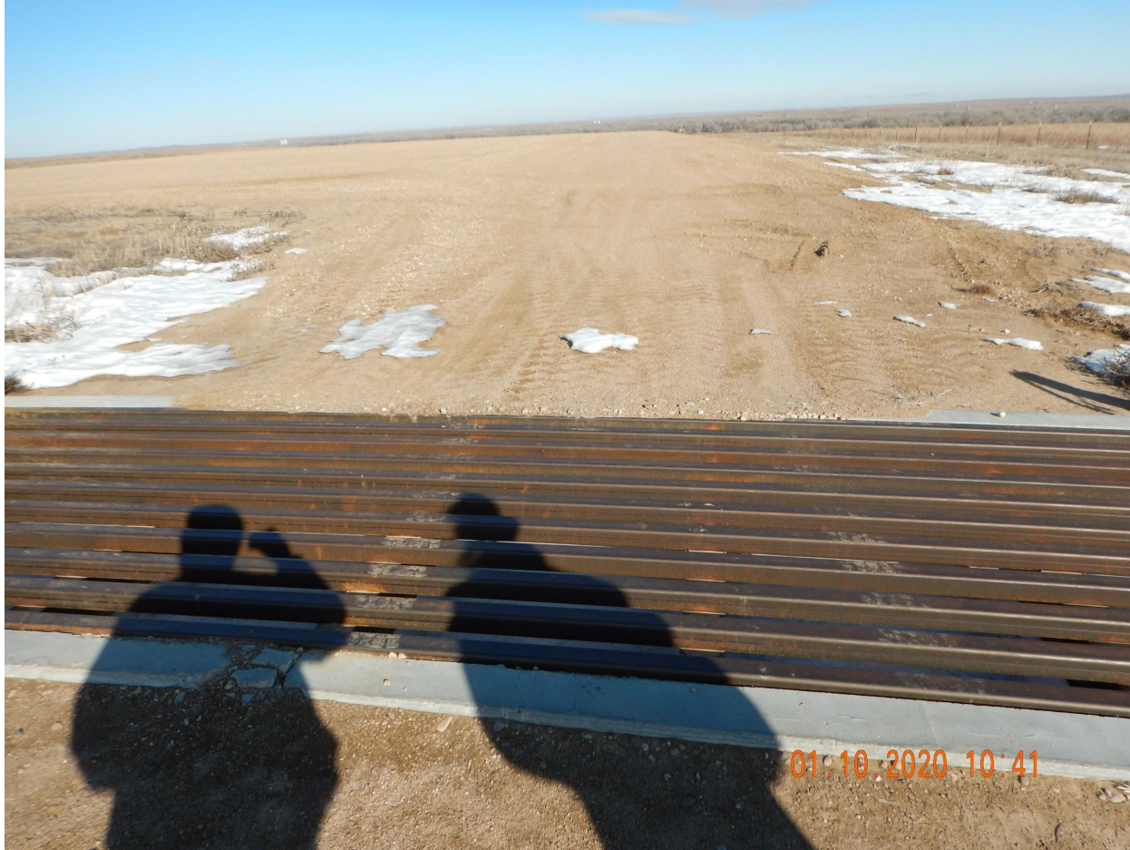
Photo 2. Photo taken from the entrance of the location, facing North. Photo illustrates another vehicle tracking device BMP.
