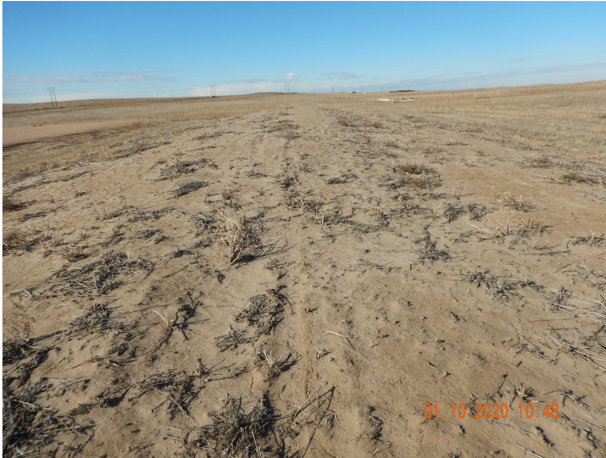
Photo 5. Photo taken from the topsoil stockpile, facing West. Photo illustrates the topsoil stockpile has not been properly stabilized and weed establishment was evident.
