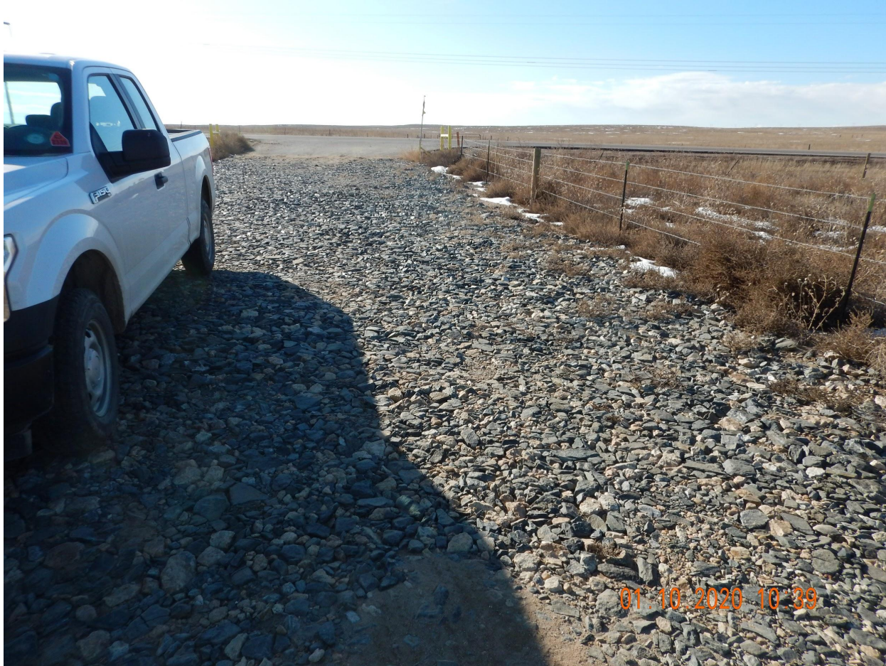
Photo 1. Photo taken from the entrance of the location off HWY 34, facing South. Photo illustrates a portion of the vehicle tracking device BMP.
