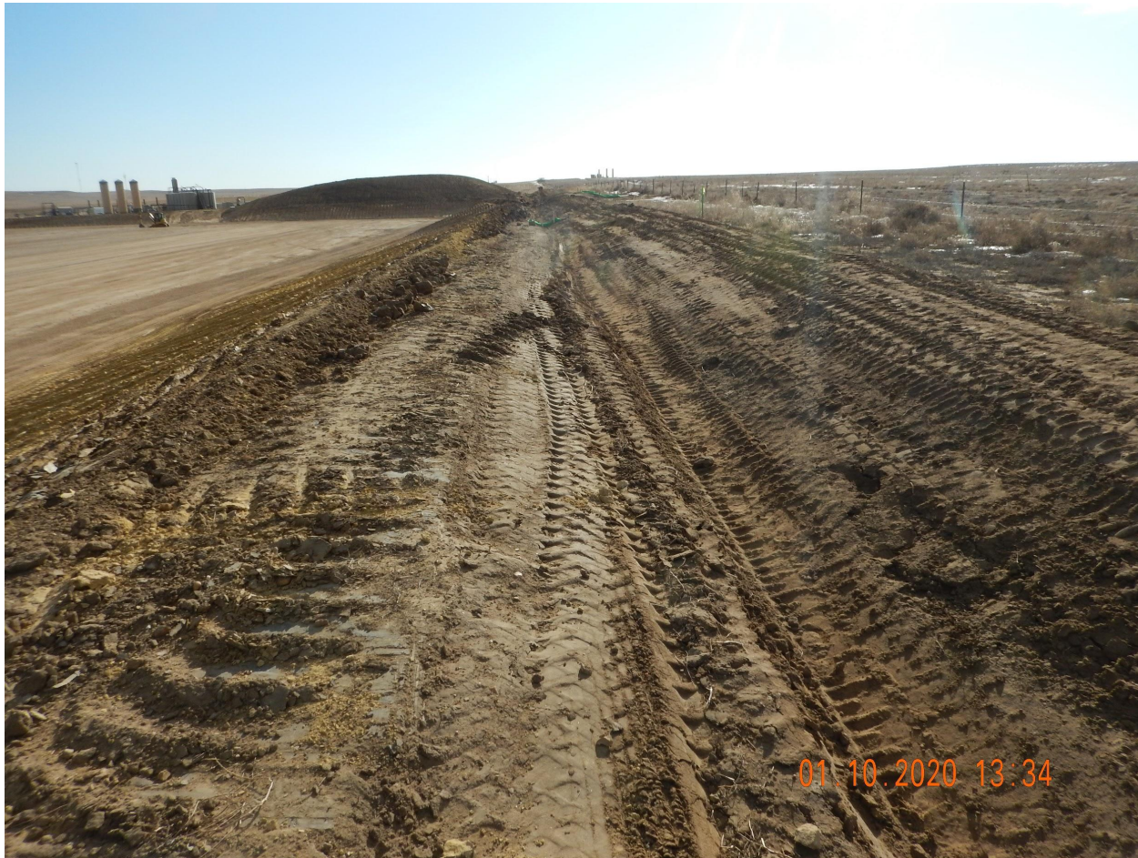
Photo 5. Photo taken from the western perimeter of location, facing South. Photo illustrates a ditch and berm BMP installed in conjunction with sediment traps and wattle check dams.
