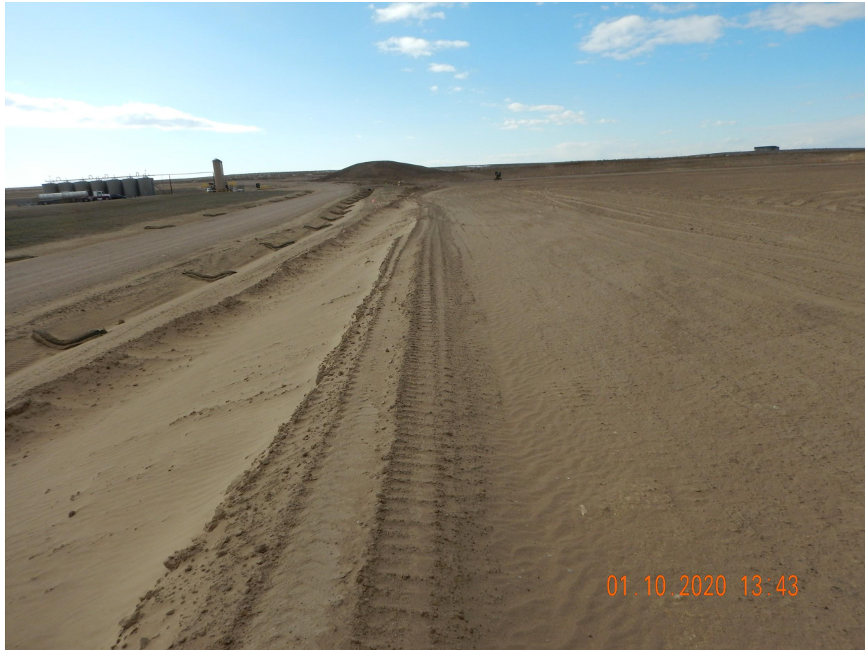
Photo 2. Photo taken from the southeastern location, facing West. Photo illustrates soil particle deposition from wind erosion along the fill slopes, filling up the ditch BMP, and off location.
