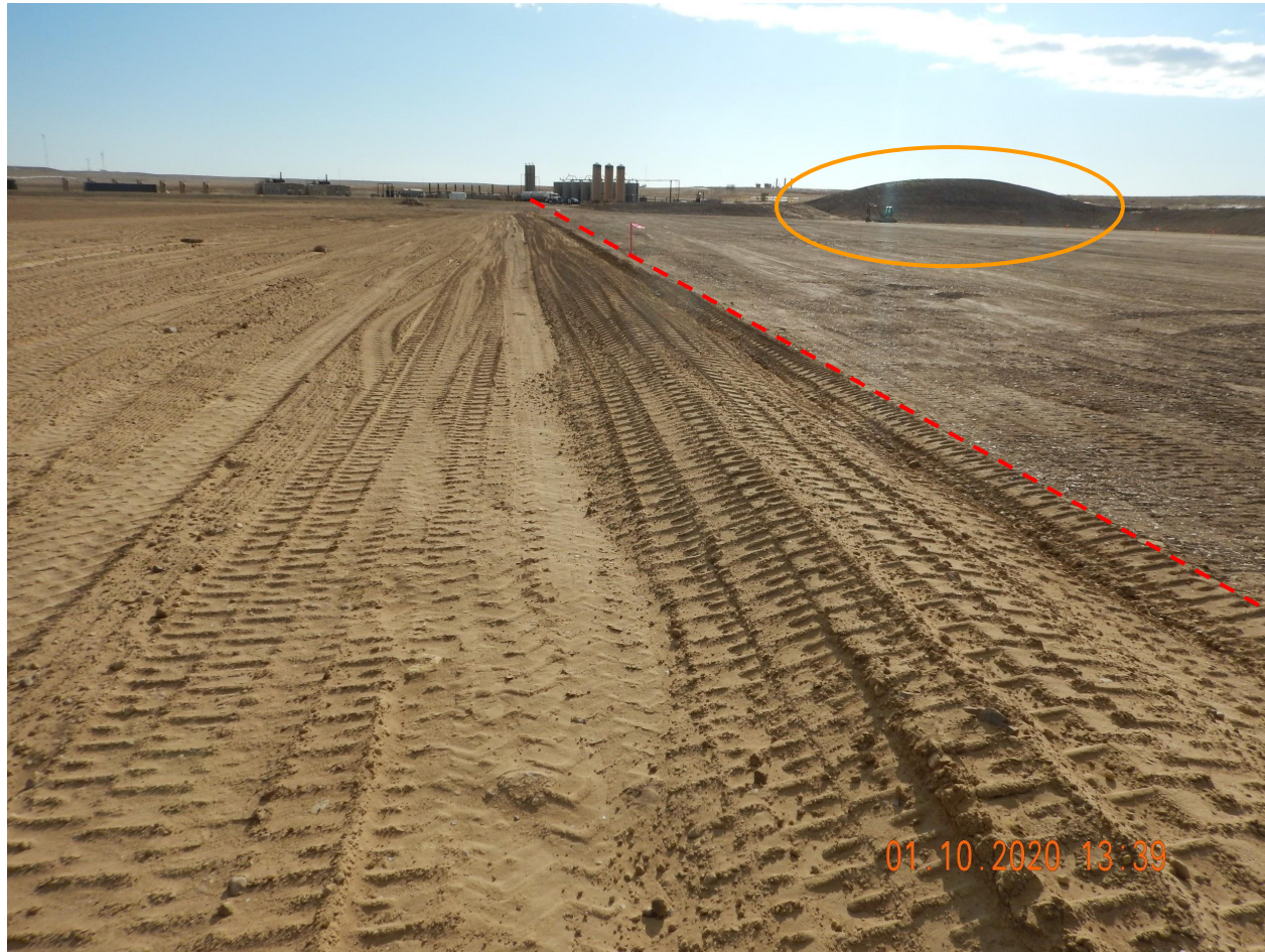
Photo 1. Photo taken from the north-central location, facing South. Photo illustrates the western portion of the location has been stabilized with gravel while the eastern portion has been left unconsolidated. Soil particle deposition from wind erosion is apparent. Also, topsoil has been salvaged and stored along the southwestern perimeter of location.
