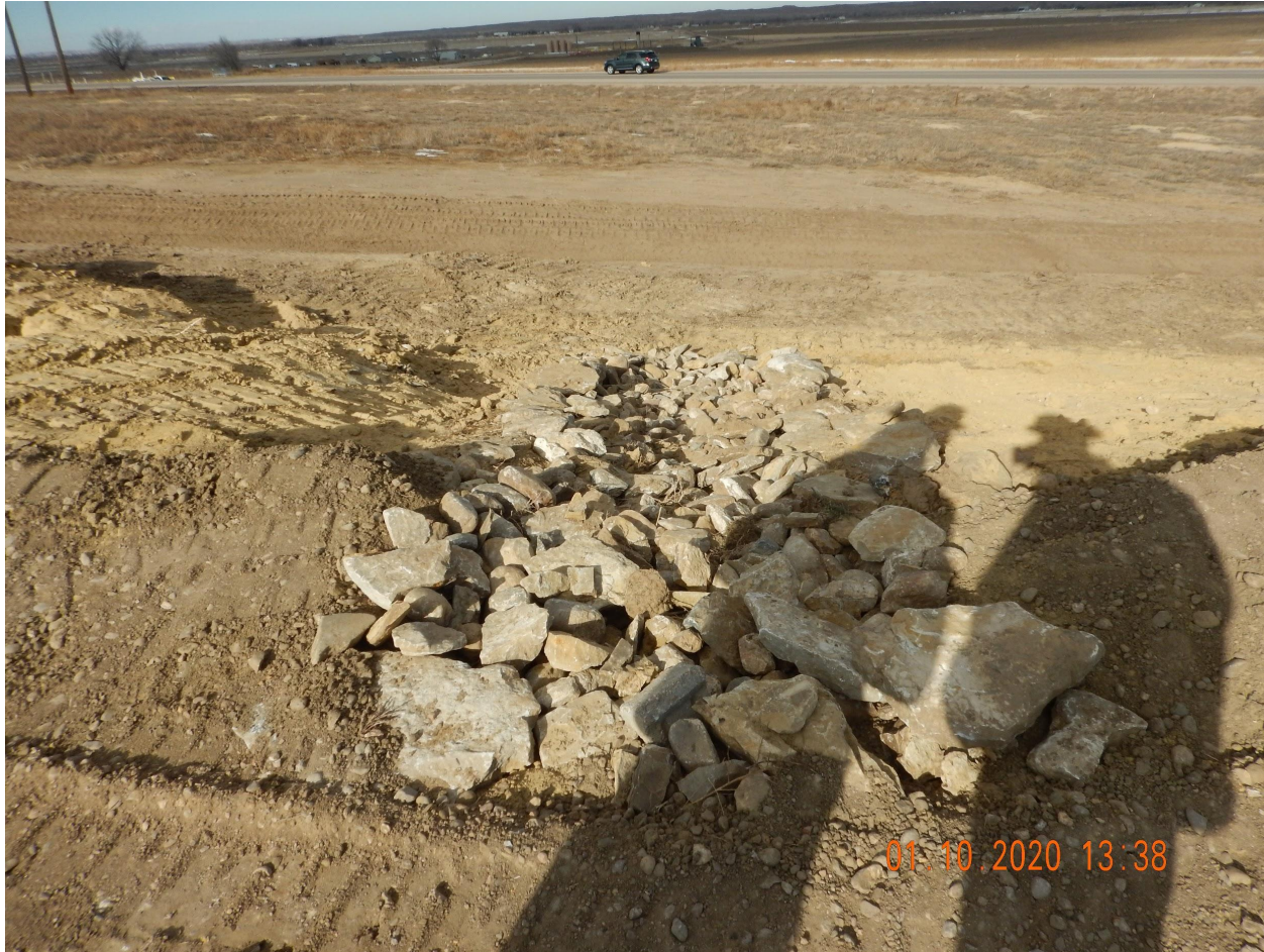
Photo 7. Photo taken from the northern location, facing North. Photo illustrates a stabilized ditch which is directed to the perimeter ditch and berm BMP and sediment trap.
