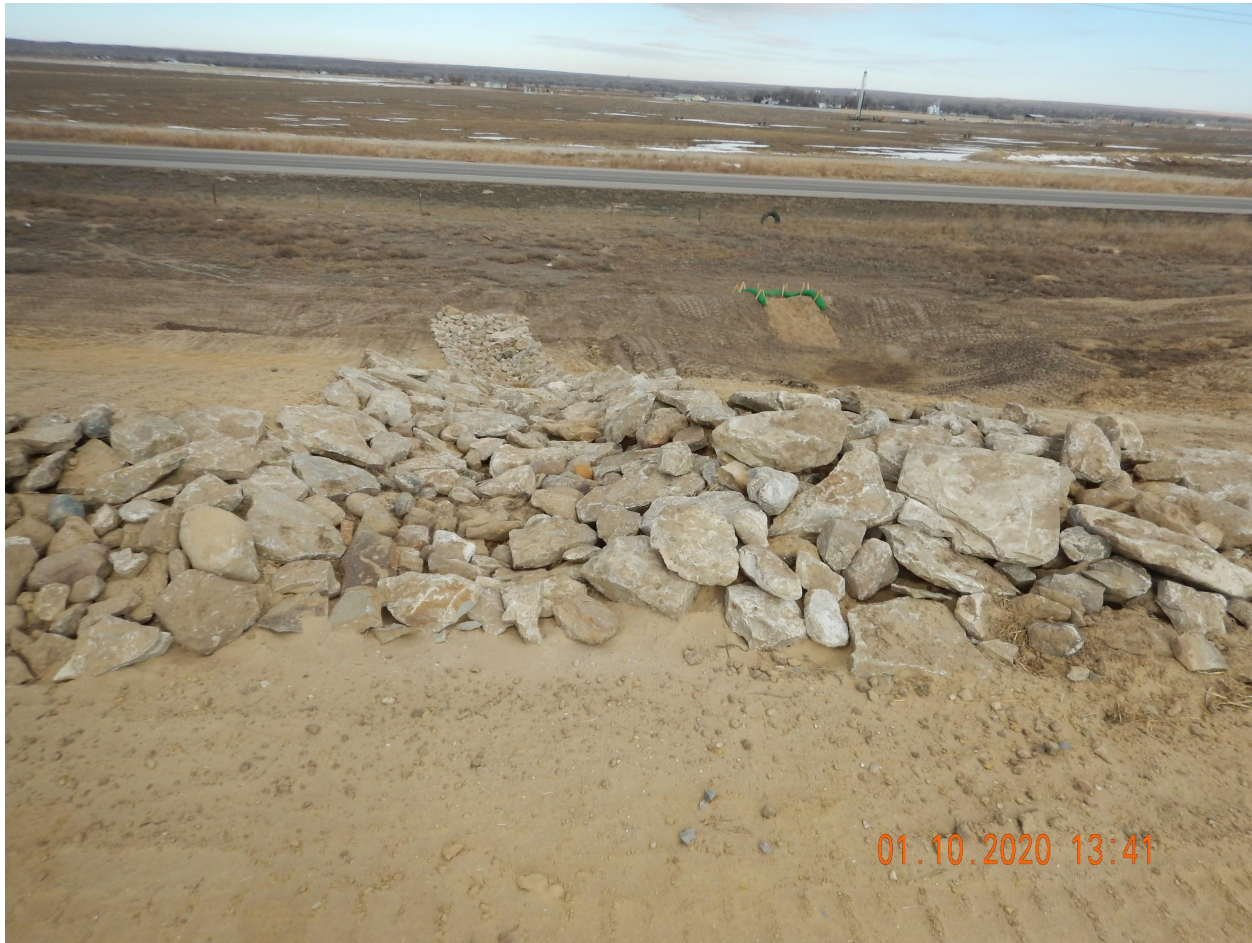
Photo 9. Photo taken from the northeastern location, facing North. Photo illustrates another sediment trap with a temporarily stabilized outlet and a stabilized ditch BMP.
