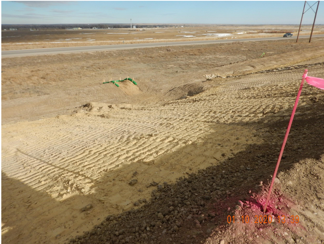
Photo 8. Photo taken from the northern location, facing Northeast. Photo illustrates one of the sediment traps with a temporarily stabilized outlet.
