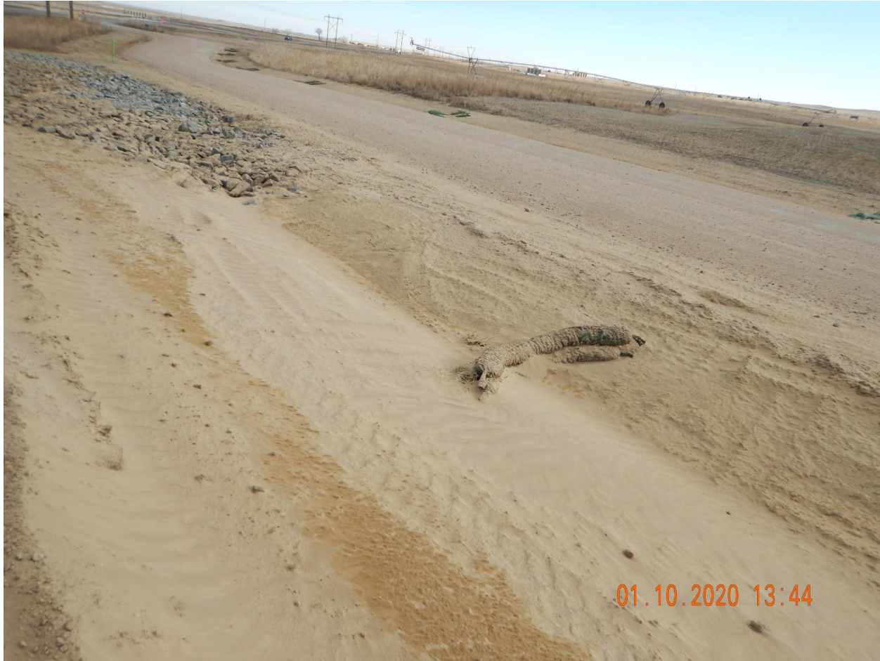
Photo 4. Photo taken from the southeastern location, facing East. See comments under Photo 2 regarding soil particle deposition from wind erosion. Note: Tackifier was observed along the southern fill slope but soil particle deposition has accumulated on top of that.
