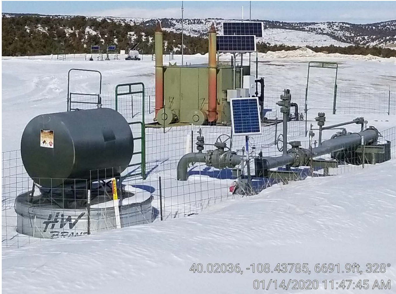
Photo 3. Separator, chemical, and pig station.
