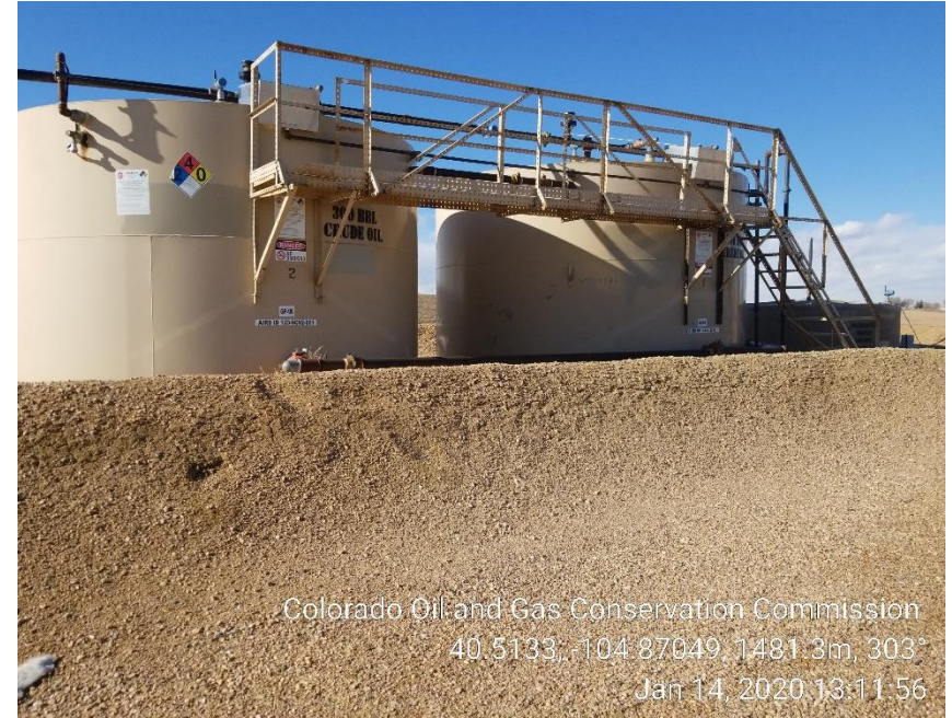
Photo 6: Tank Battery
