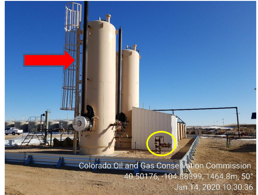
Photo 8: Disconnected heater treater/unused risers
