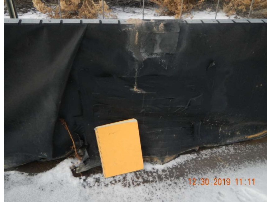
Photo #4 – Patch in disrepair and the 2 – 3-inch residual staining ring located on the west side of the tank battery.
