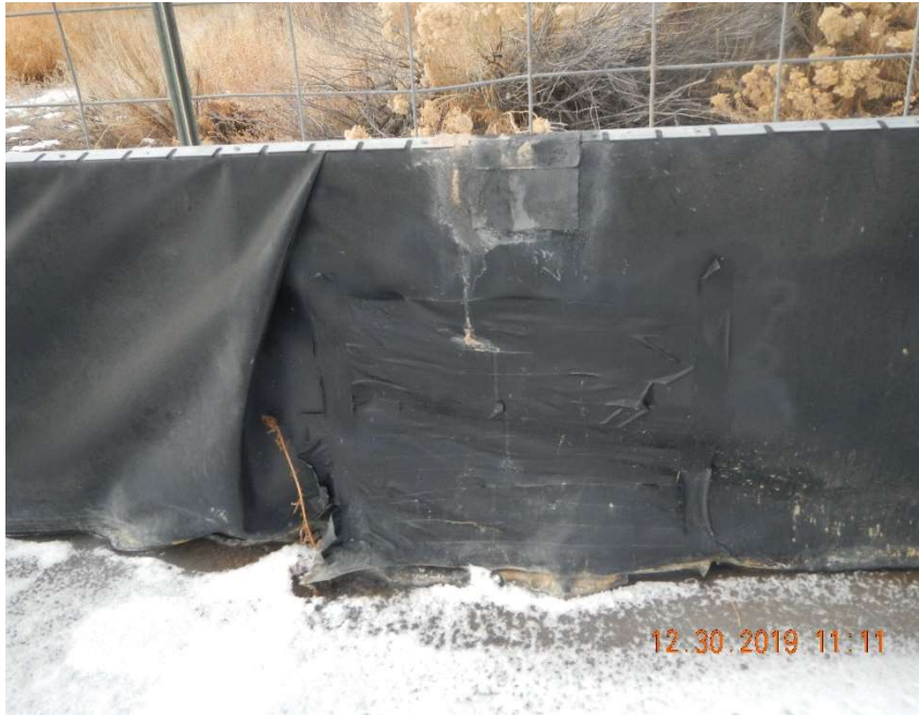
Photo #5 - Patch in disrepair and the 2 – 3-inch residual staining ring located on the west side of the tank battery.
