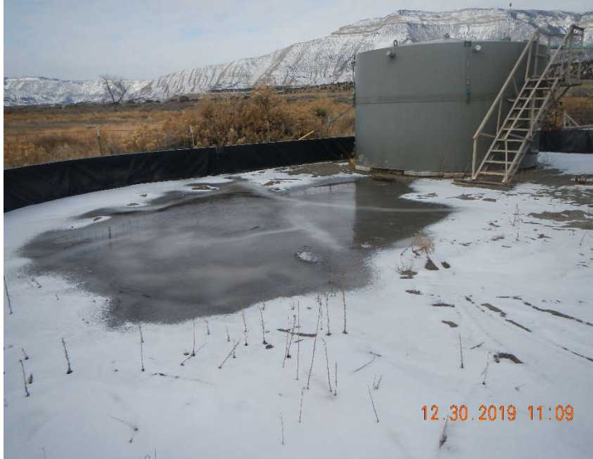
Photo #3 - Frozen fluids within the tank battery secondary containment.
