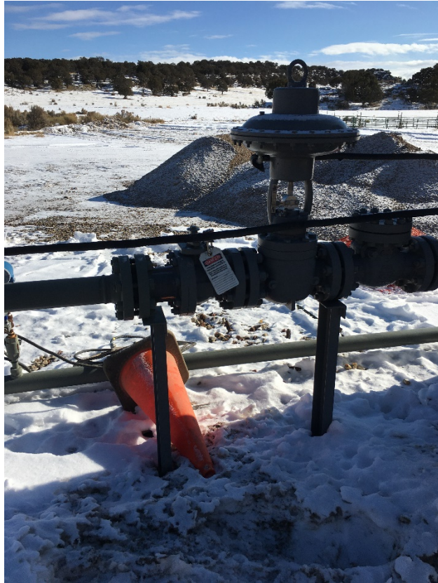
Sales line locked out and tagged out
