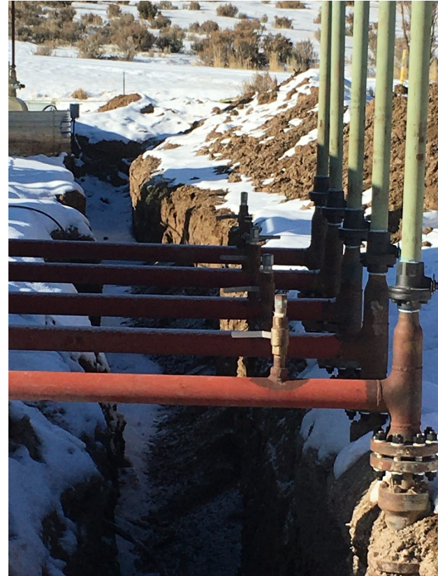
Dump line running in trench to tank battery
