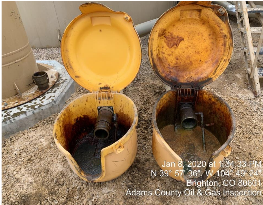
Photo#9 Bullplugs Missing/Right bucket needs emptied out
