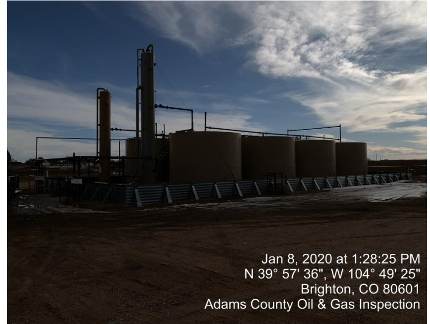
Photo#2 (6)Production Tanks/(2) Produced water tanks/(2)VRTs
