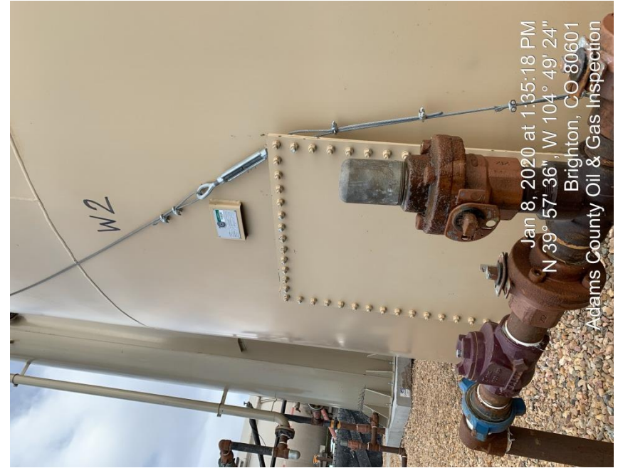
Photo#12 Balon valve leaking
