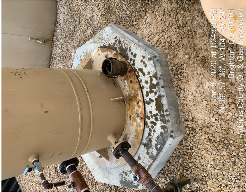
Photo#11 VRT leaking from PRV
