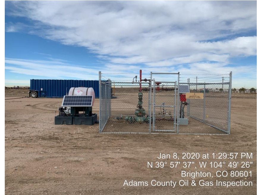
Photo#4 Wellhead/Chem tank OPS 2501V Oil soluble Paraffin Solvent
