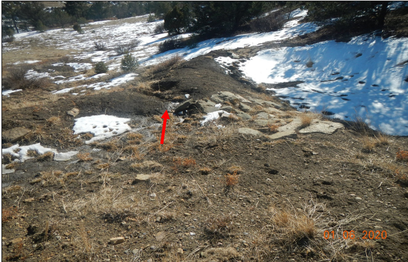
Photo 6. An erosion channel has developed which is preventing stormwater from entering the sediment trap. This is located at the south side of the location.
