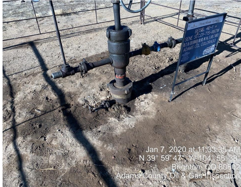
Photo#5 Corrective Action: Stained Soil needs Cleaned Up
