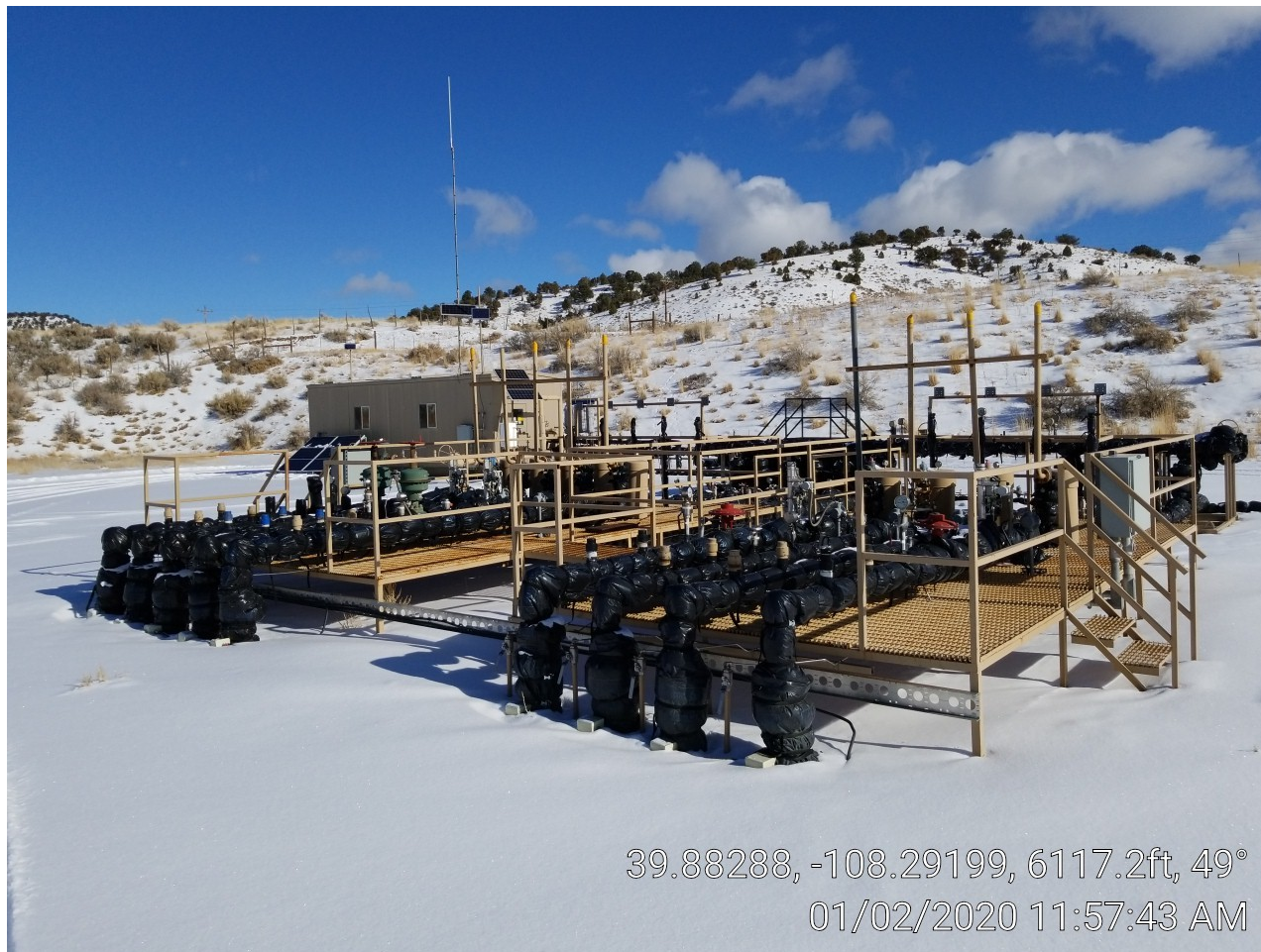
Photo 3. Well manifold.
