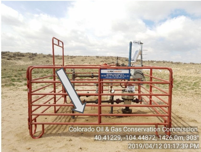
Photo #1 NHF 13-9 (05-123-20921) Wellsite Temporarily Abandoned | TA Stained soil at wellhead perimeter prior insp.
