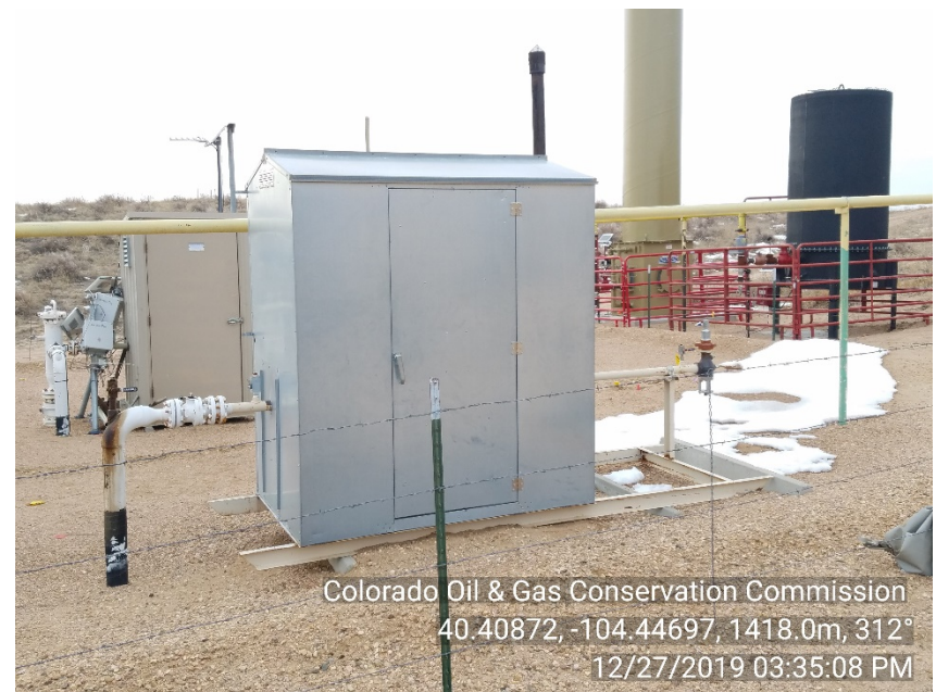
Photo #6 NHF 13-9, 24-9 Battery site Unused Equipment Gas meter run, riser: Company states plans to re-use
