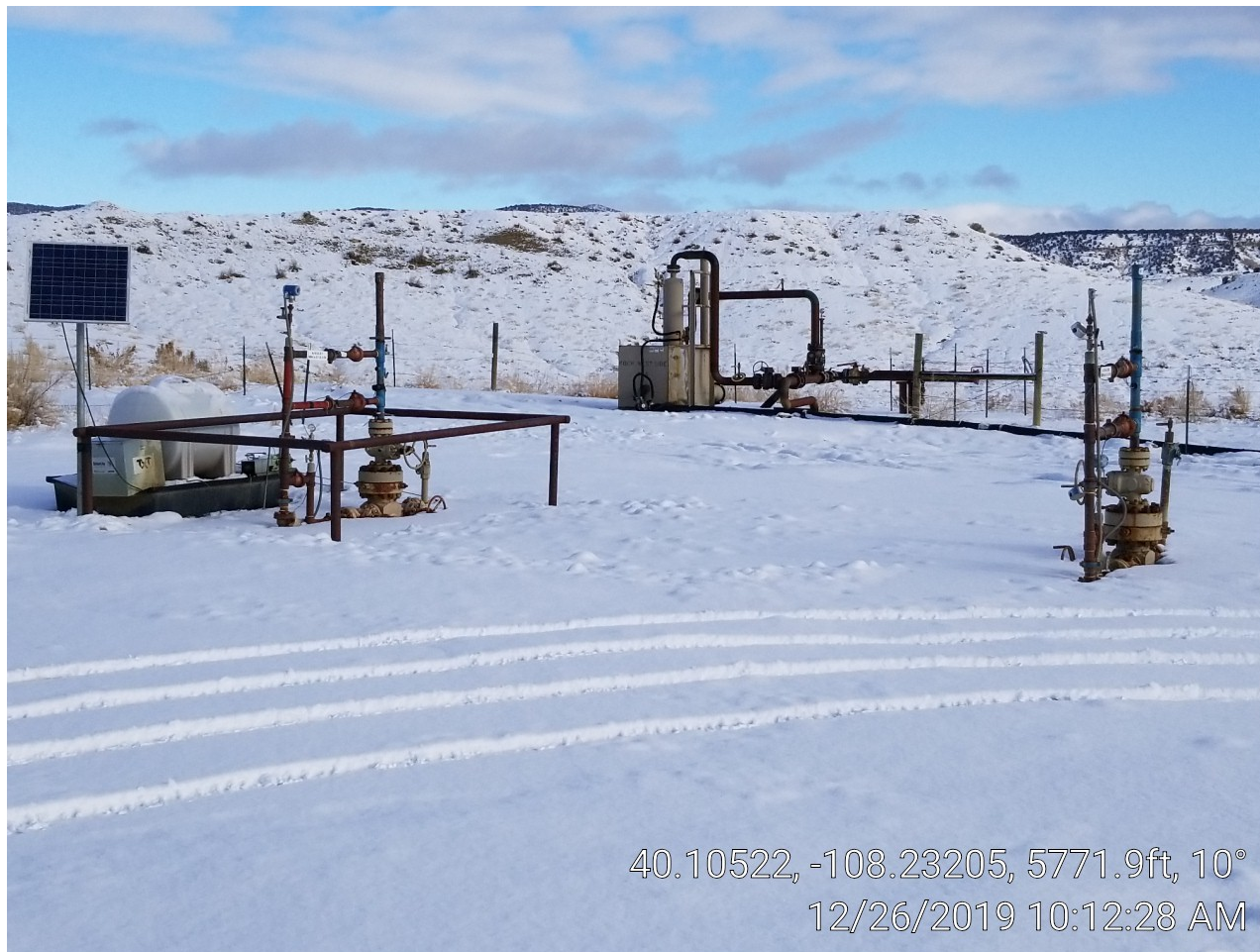
Photo 2. Well heads & pig station.
