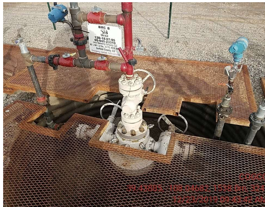
Well heads missing wildlife escape boards.
