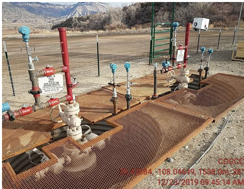
Well heads missing wildlife escape boards.
