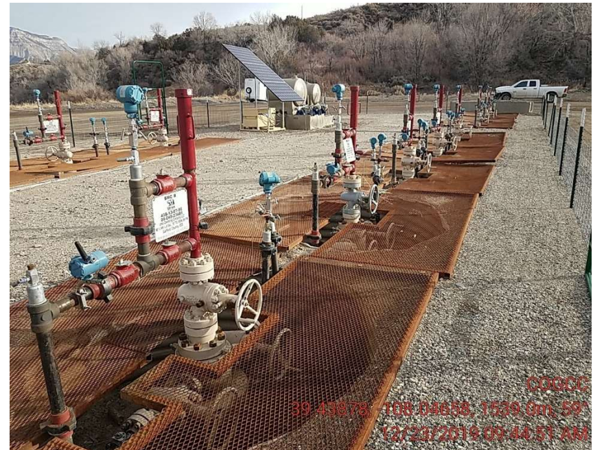
Well heads missing wildlife escape boards.
