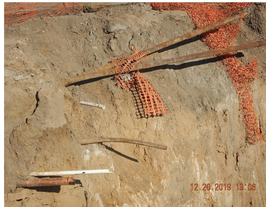
Cut ends of flowlines exposed in excavation (in north wall).
