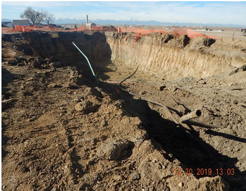
View of excavation; flowlines exposed in ground and walls (view west).
