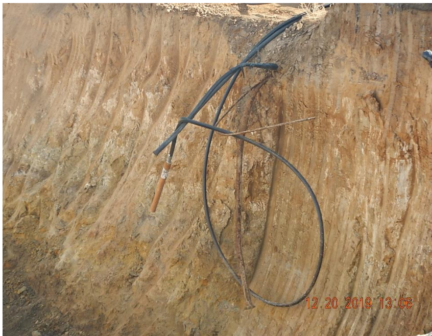
Cut ends of flowlines exposed in excavation (in south wall).
