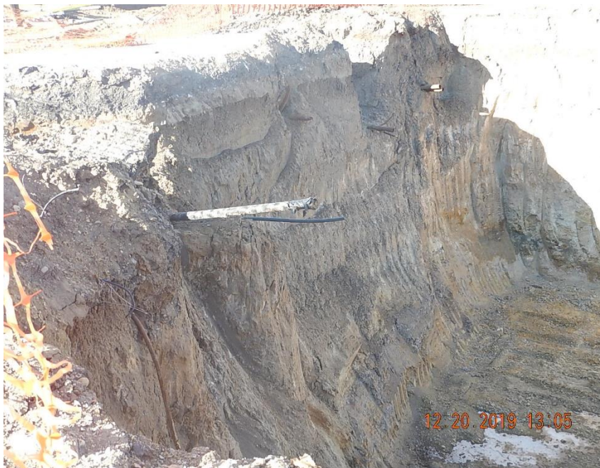
Cut ends of flowlines exposed in excavation (in west wall).
