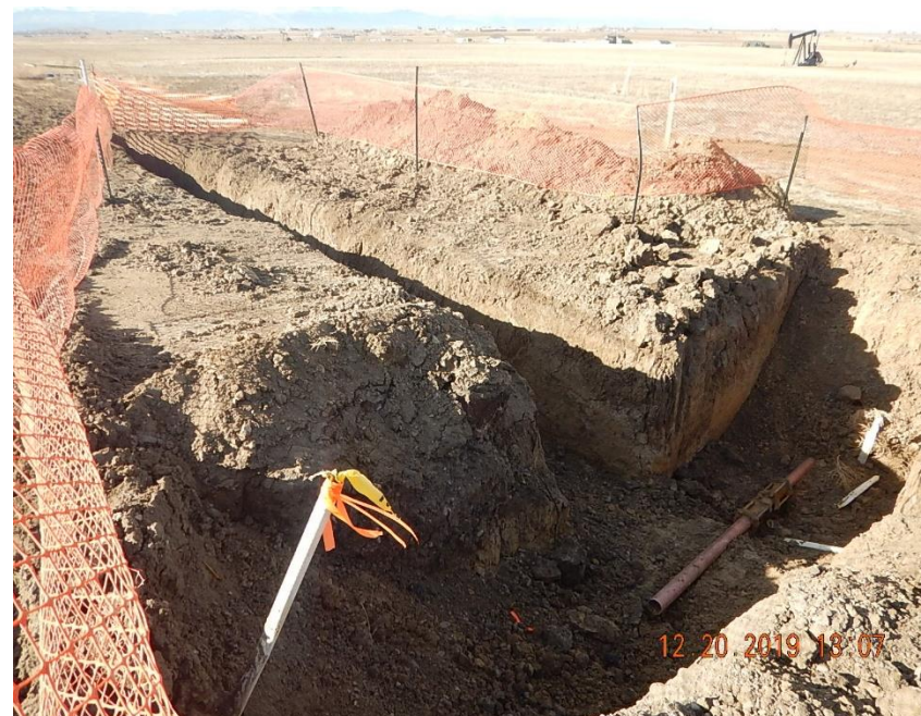
Cut ends of flowlines exposed in trenching/ excavation recently completed approximately 30' north of the north wall of the primary excavation; ends open to atmosphere.
