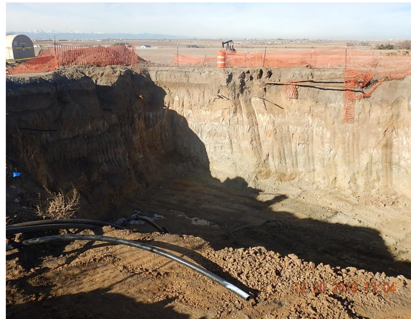
Cut ends of flowlines exposed in excavation ( view to NW).
