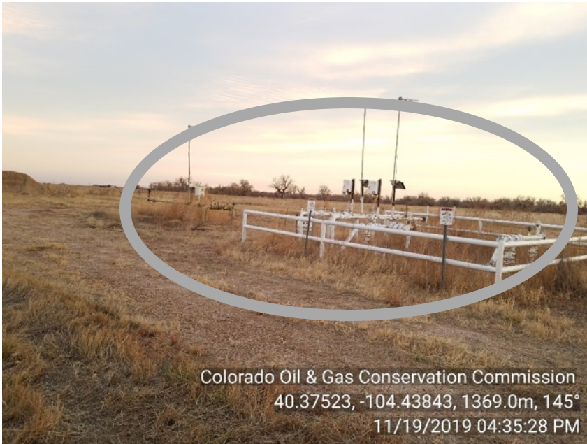
Photo #1 DOW 32-28 Battery site Abandoned | Most equipment removed Reclamation progressing Unused Gas meter runs prior insp.
