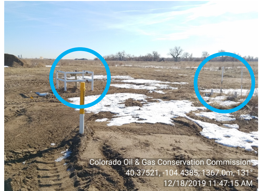
Photo #2 DOW 32-28 Battery site Abandoned | Most equipment removed Reclamation progressing Marked & capped risers: 3
