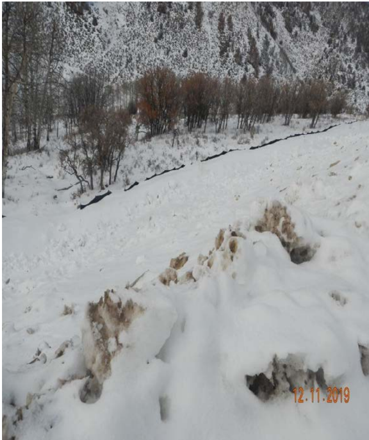
Photo#2: Silt fence in disrepair along site perimeter.
