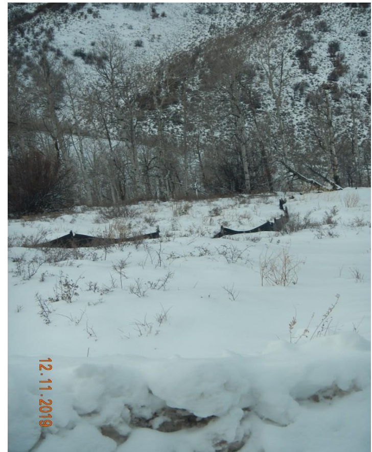
Photo#3: Silt fence in disrepair along site perimeter.
